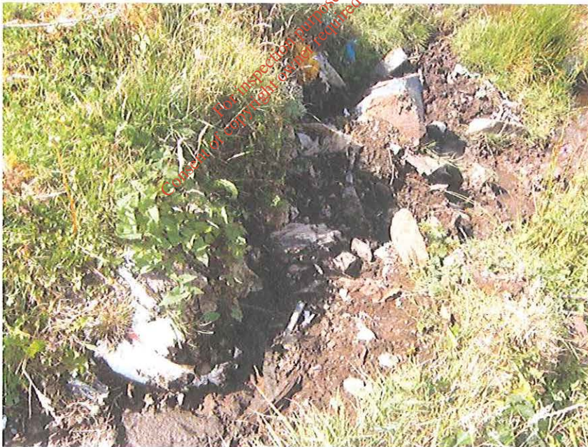
Photo No. 2 – Waste protruding from waste body.
