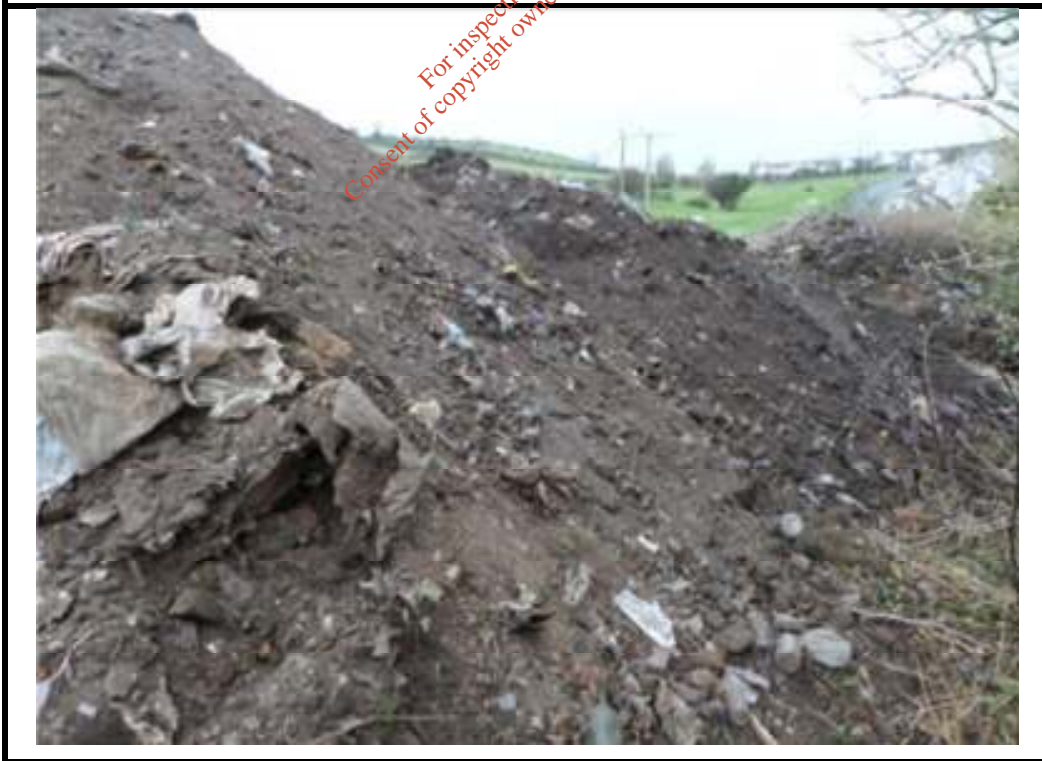
Photograph 15: Waste Contained in Trial Hole 14 (TH 14).
