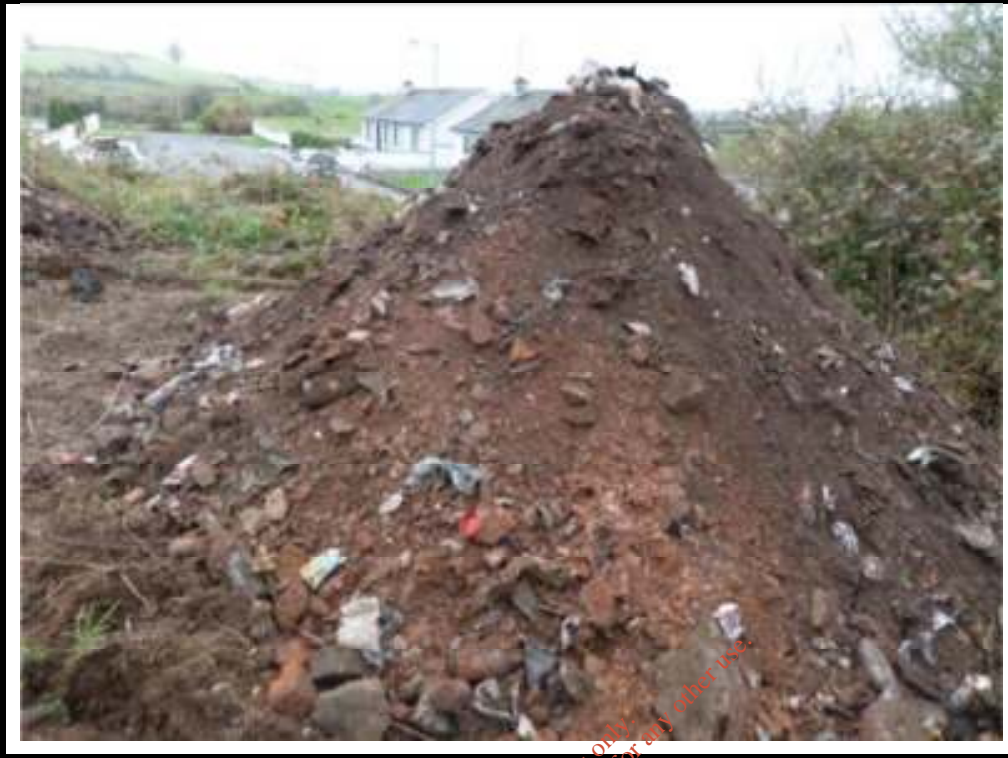
Photograph 8: Waste Contained in Trial Hole 7 (TH 7).
