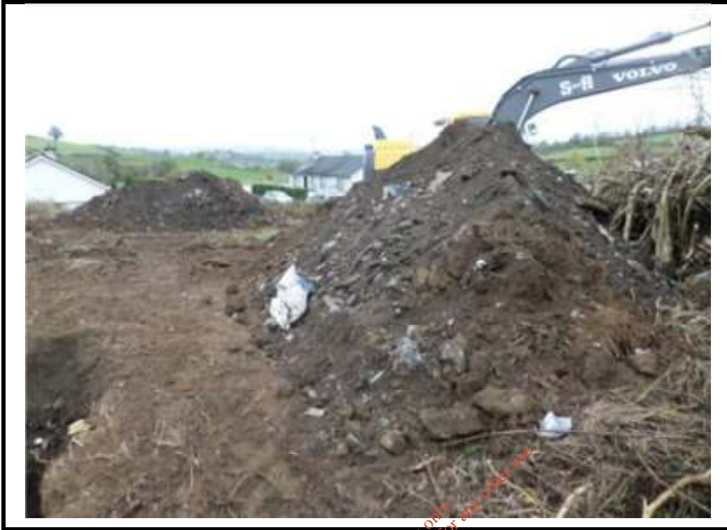
Photograph 14: Waste Contained in Trial Hole 13 (TH 13).
