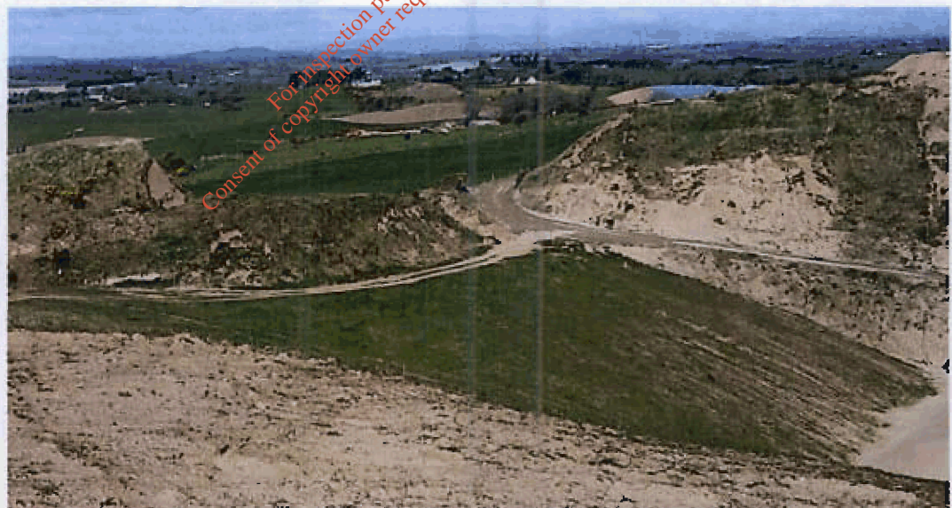
Restoration work undertaken on southern elevation
