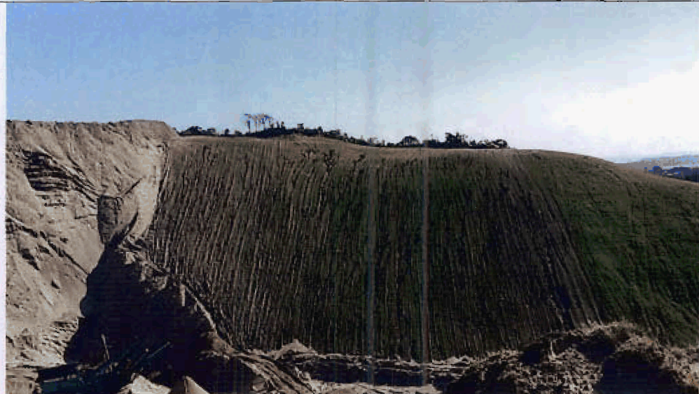
Restoration work undertaken on part of the eastern elevation
