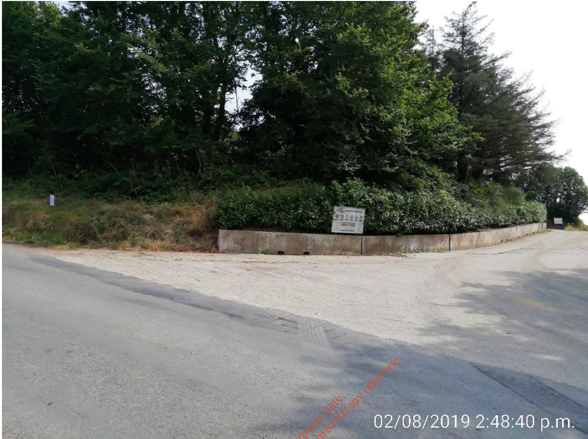
Photo 4: View 3 of erected Site Notice located to left of the site access entrance. Photo taken from road (L-7003-1) facing southeast towards site entrance.
