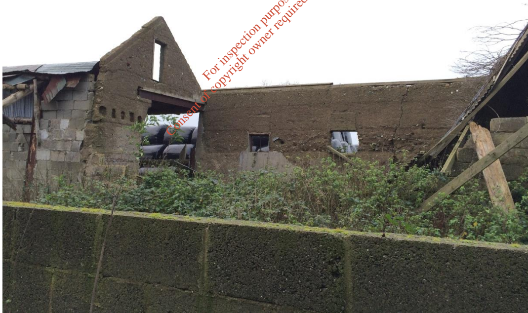
Plate 13.11 – Buildings at the site of the post medieval farmstead, facing northwest
