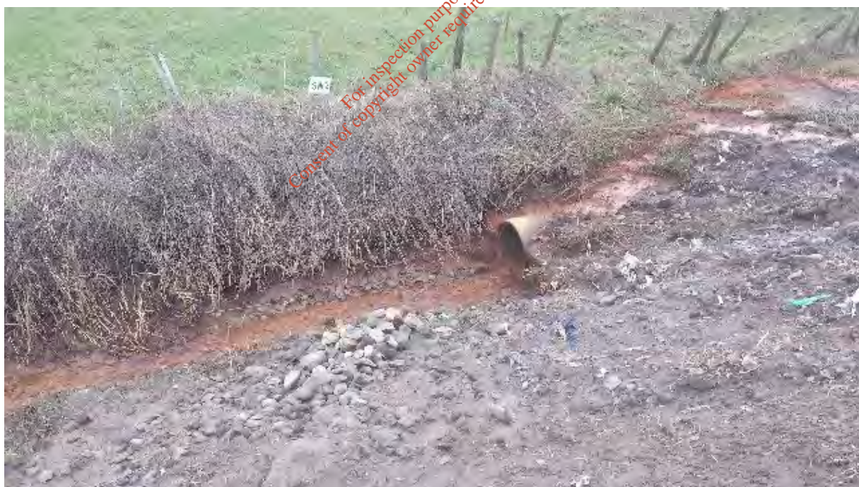
Figure 8.9 Leachate Impact within Northeastern Boundary Drain pre-restoration
