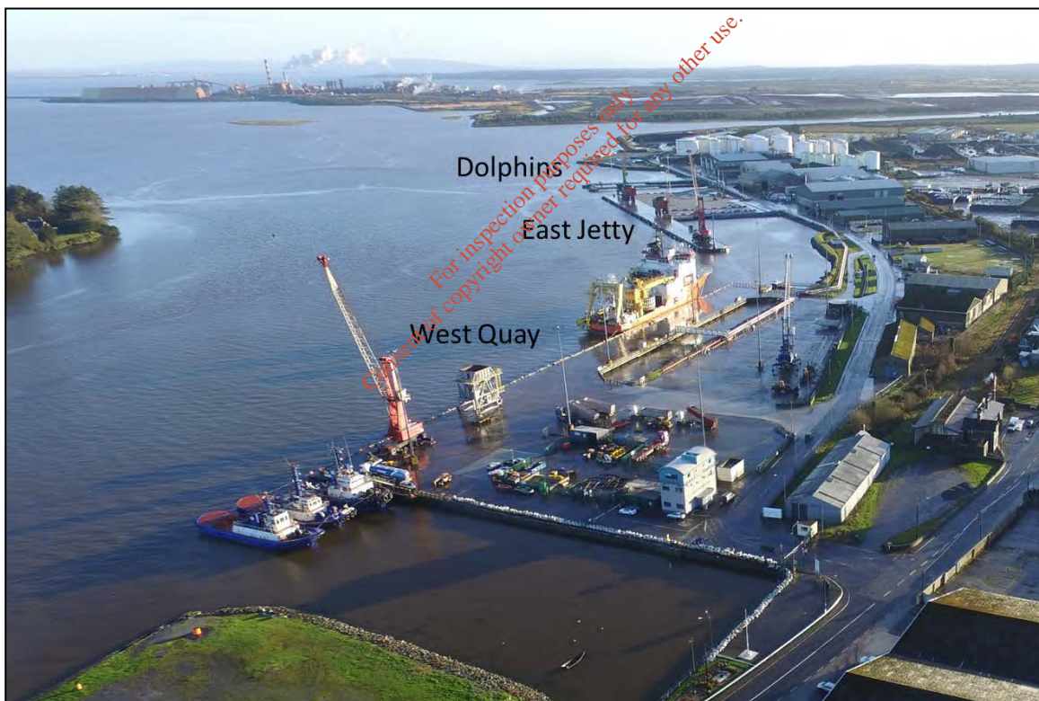
Photograph D.1-3- An Aerial View of Foynes Harbour
