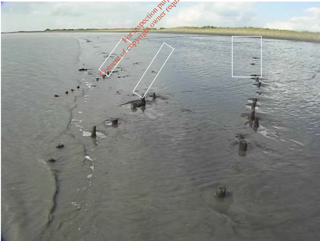
Fig 2.5 Soft estuarine mud overlaying posts on mid / upper foreshore 2002
