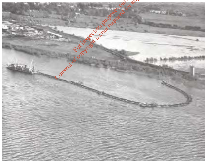
Photograph C.1-1- Dredged Spoil being pumped ashore 1956
