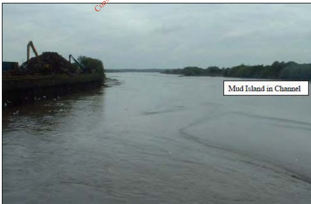
Photograph D.1-8- Picture showing large build of silt at the Entrance Channel to Limerick Dock where the river widens
