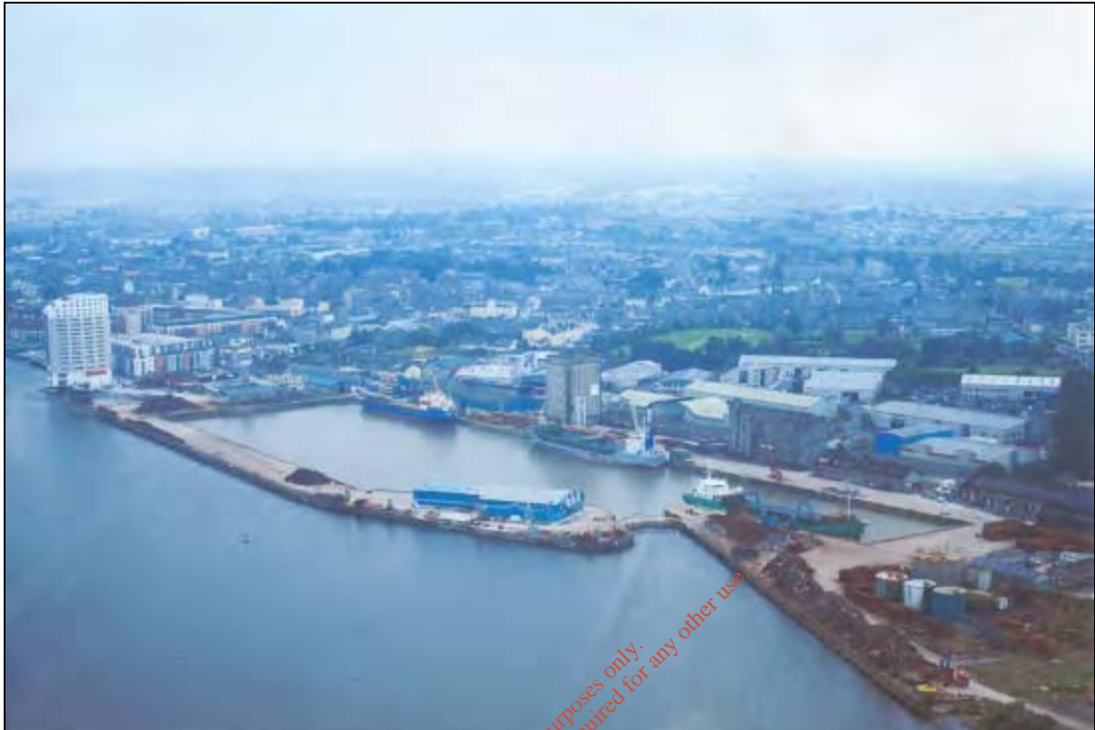
Photograph D.1-2- Ted Russell Docks today looking upstream showing the enclosed Dock and the Approach Channel
