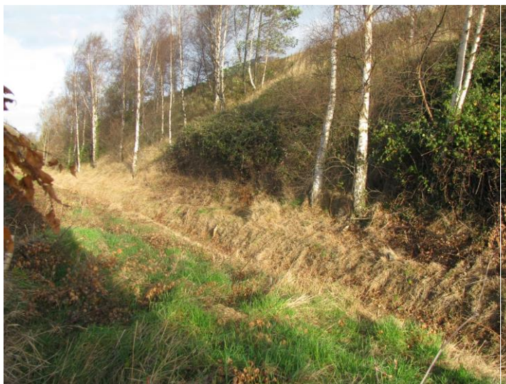
Insert 1.6. – M50 Toe drainage
