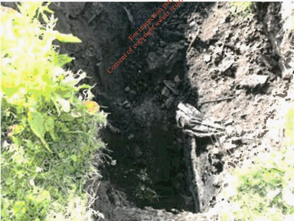
Photo 4- Trial pit excavations showing buried mixed waste beneath
