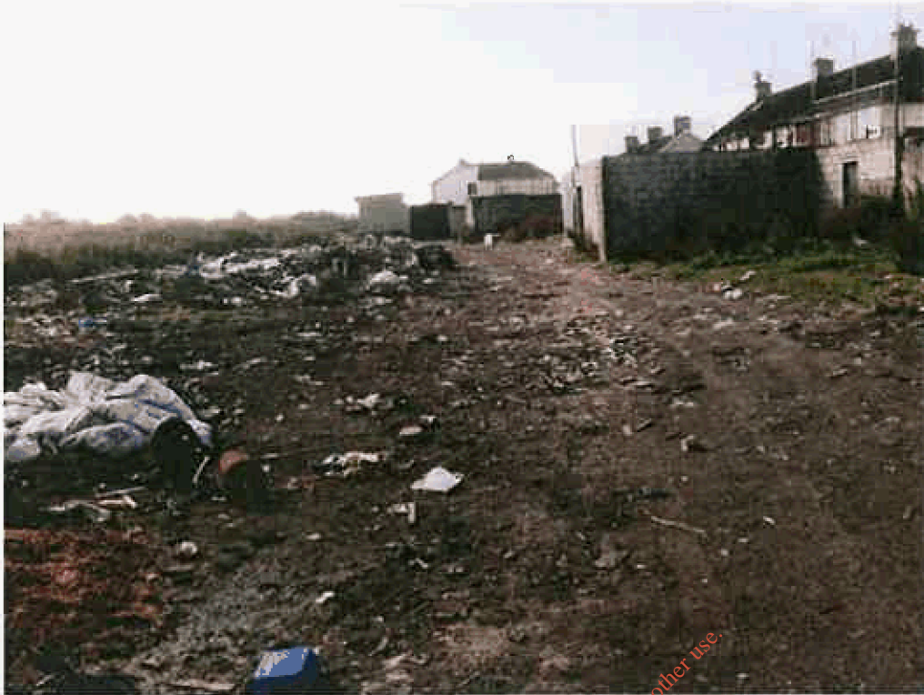
Photo 1 - Access road between rear of houses and the landfill
