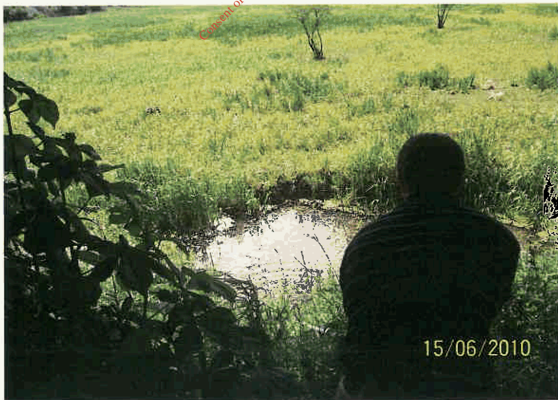
SW 2 - Drain in Back Field
