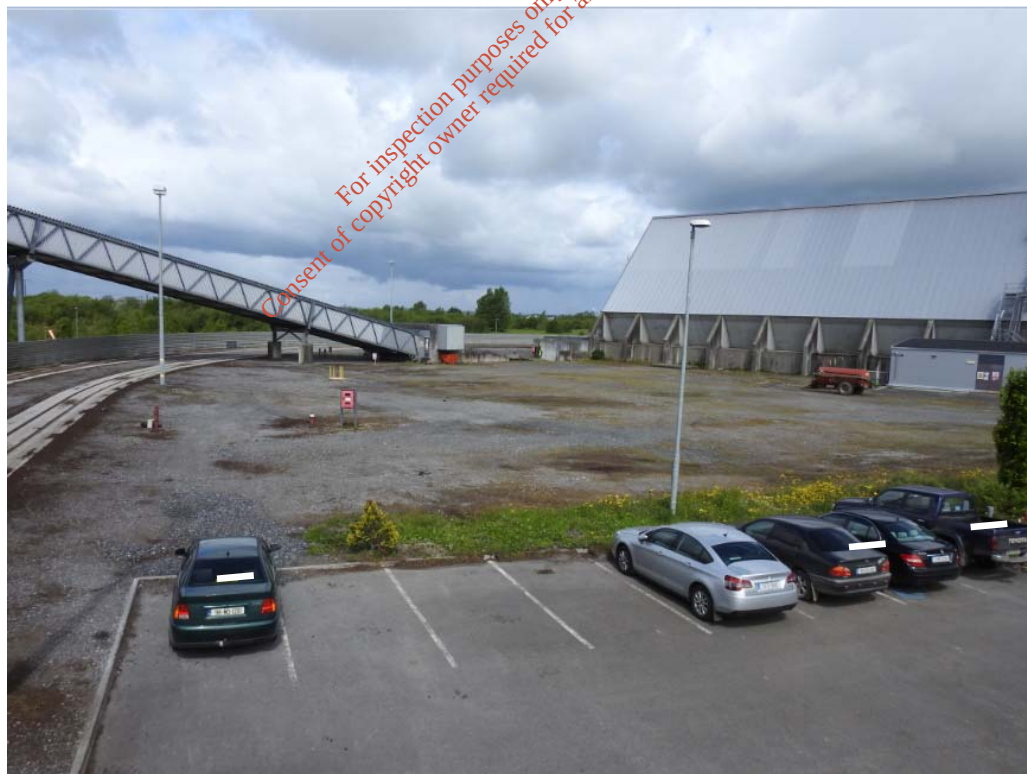
Figure 4-8: Ground view of Biomass Storage Slab A
