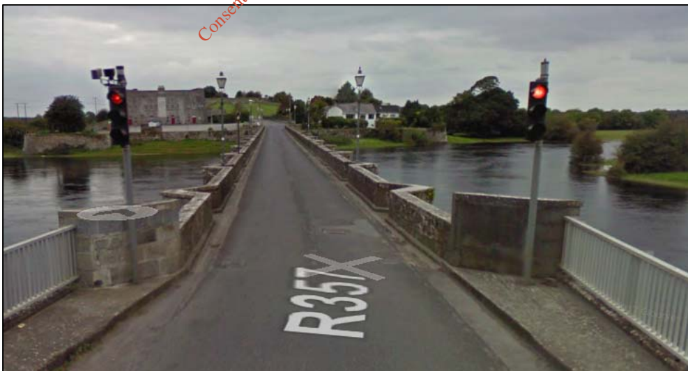
Figure 12-8: Shannonbridge bridge crossing
