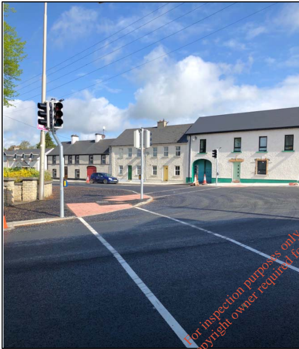
Figure 12-12: New signalised junction in Cloghan
