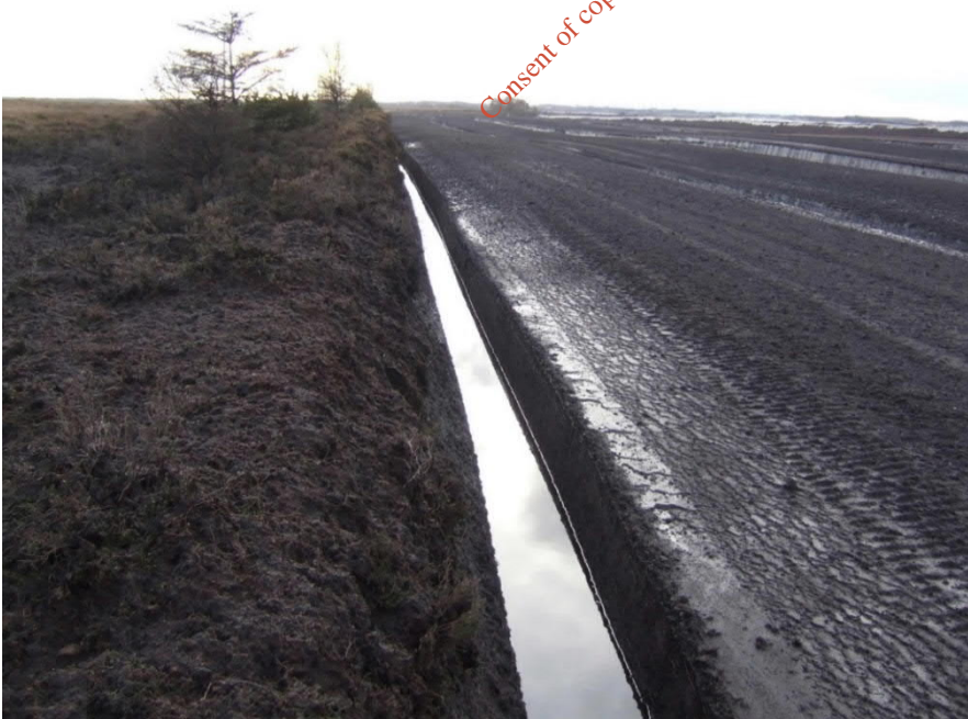
Figure 35: View of drain at edge of high bog at northeast end of Cornafulla Bog (looking southeast). Note wet peat thrown up on edge of high bog from recent drain clearing
