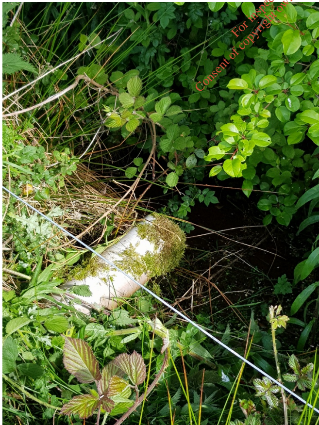
Photograph 2: Pipe (Site inspection 22/5/19)
