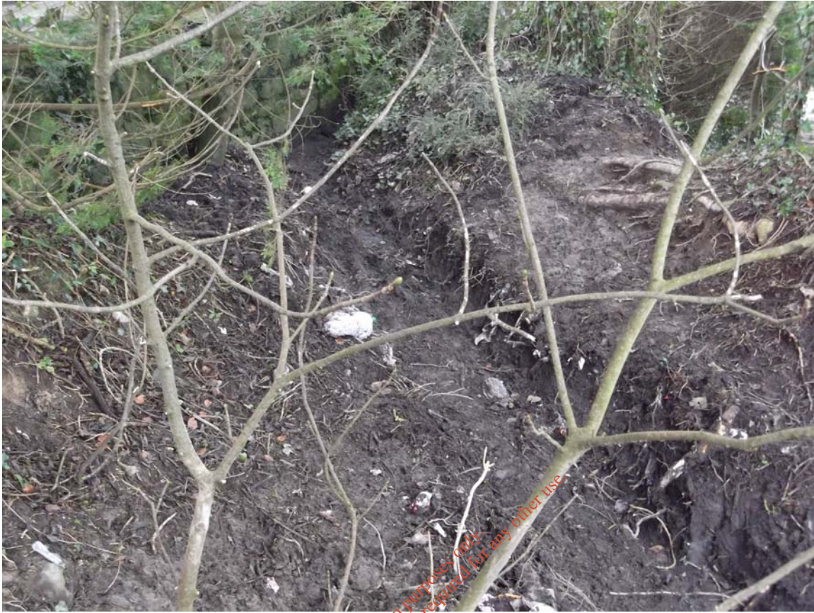
Figure 2: the outlet from the site is shown in the top centre of the photo. The fall in the drain is back towards the site itself and towards a sump constructed in the western boundary area of the landfill.
