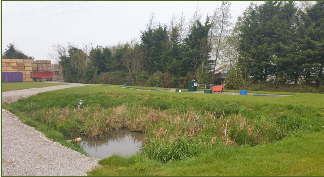
Plate 2 Example of settlement pond incorporating constructed wetland for water treatment at Vegetable Washing Plant
