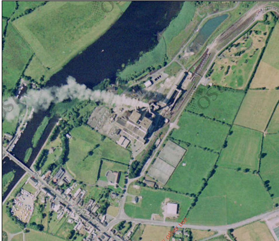
Plate 12-1 Aerial view of Lanesborough Power Station in 2000
