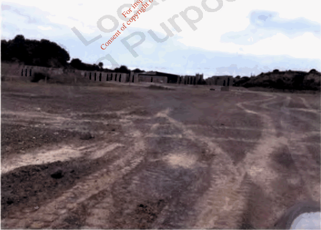
Fig. 2 – View of northern extent of application site area with existing block curing shed proposed to contain a waste inspection and quarantine facility in background
