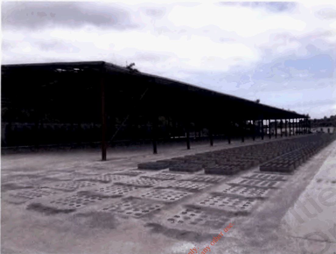
Fig. 3 – Image of existing concrete block curing shed to the north of subject site
