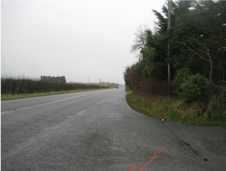
Photograph 1: Site Access Visibility Sightline to South
