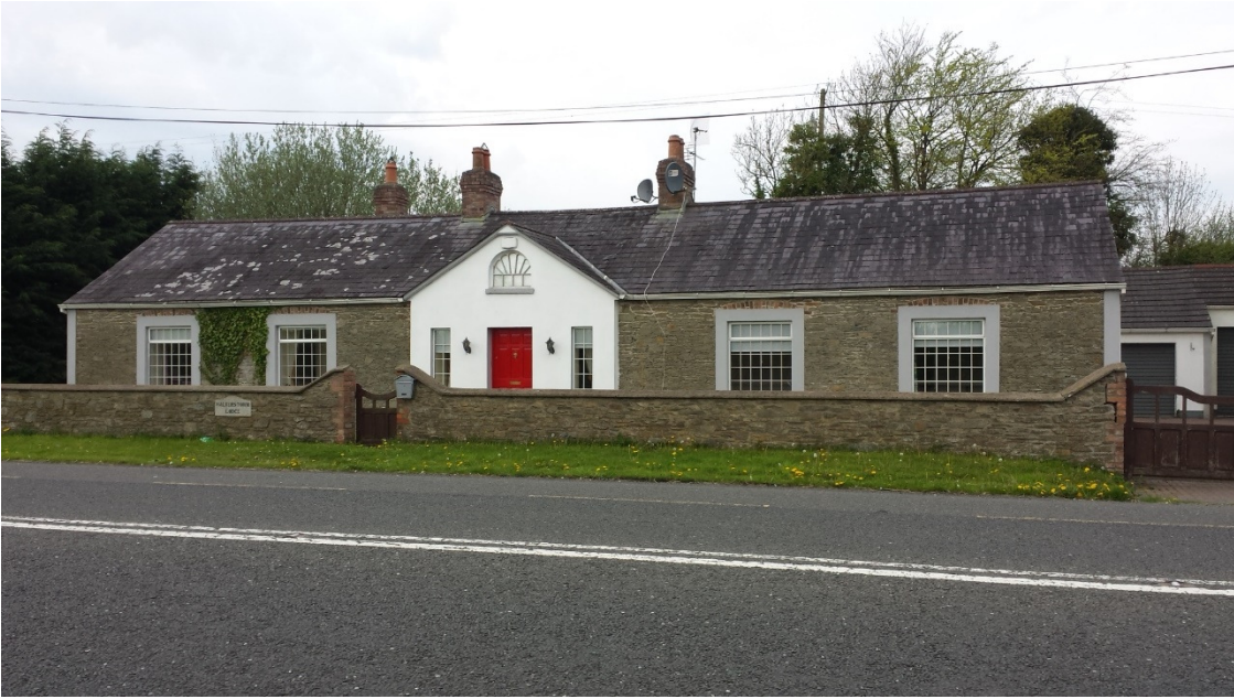
Plate 12-1: Structure 1 looking south-west.
