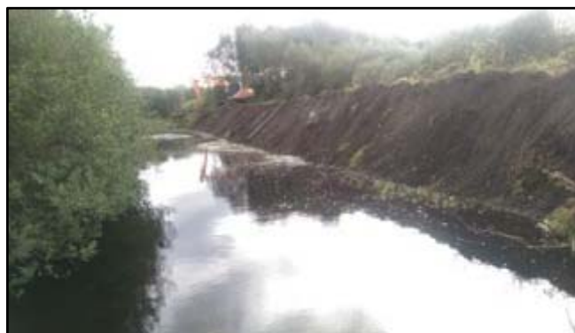
Plate 16: Detail of Drain 4 (Section F) being excavated.
