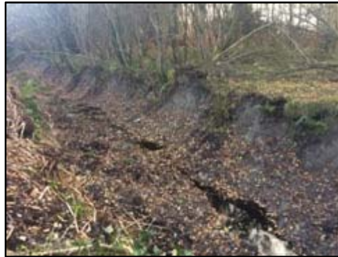
Plate 15: View of south facing section of Drain 3 Section E.
