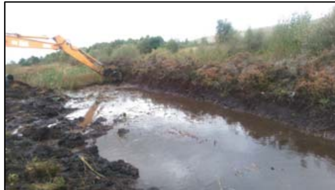
Plate 12: Detail of the western end Drain 2 being cleaned.
