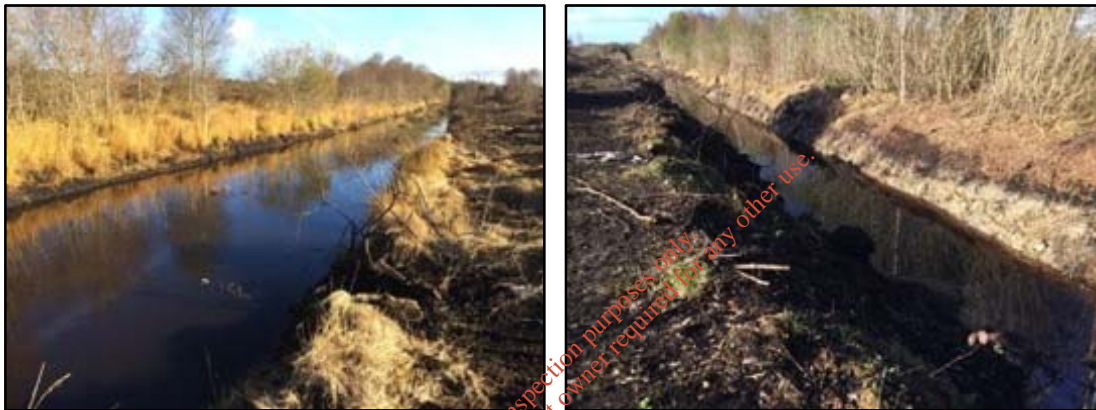
Plates 17 & 18: Drain 4 (Section G) from the west and east.
