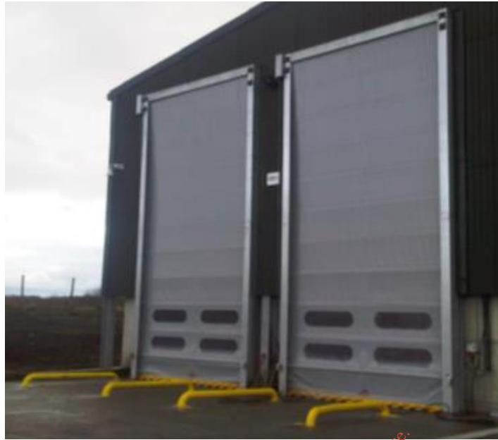
Figure 3.5: Waste Receiving Doors at the Existing Facility
