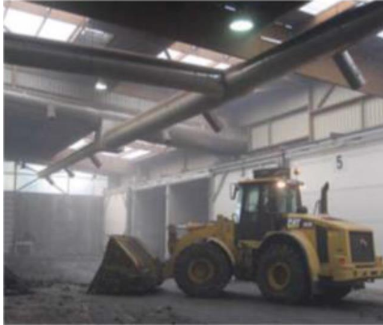
Figure 3.7: Loading of Dry AD Tunnels
