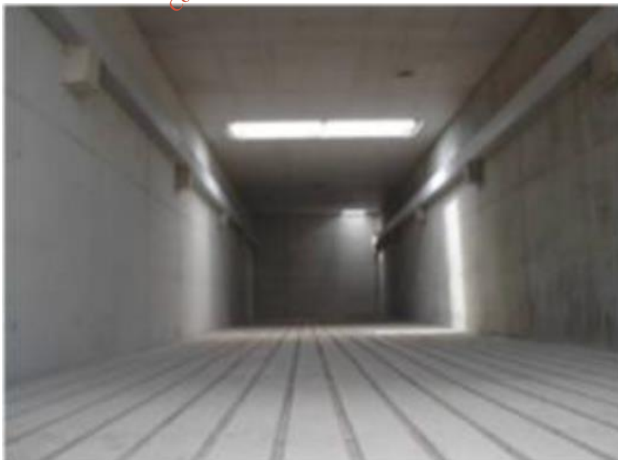
Figure 3.4: Typical Composting Tunnel with Spigot Floor
