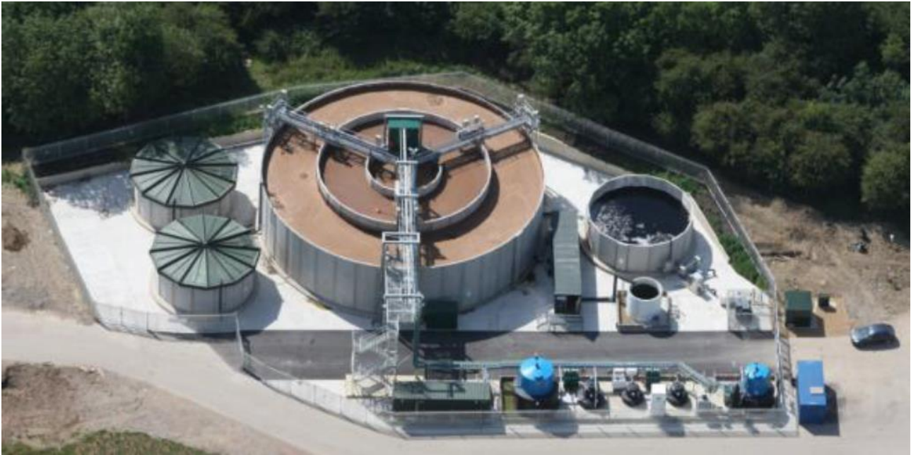
Figure 4.2: Similar Concentric Tank arrangement at Bletchley Leachate Treatment Facility, Buckinghamshire, UK. (Photograph provided for illustrative purposes)
