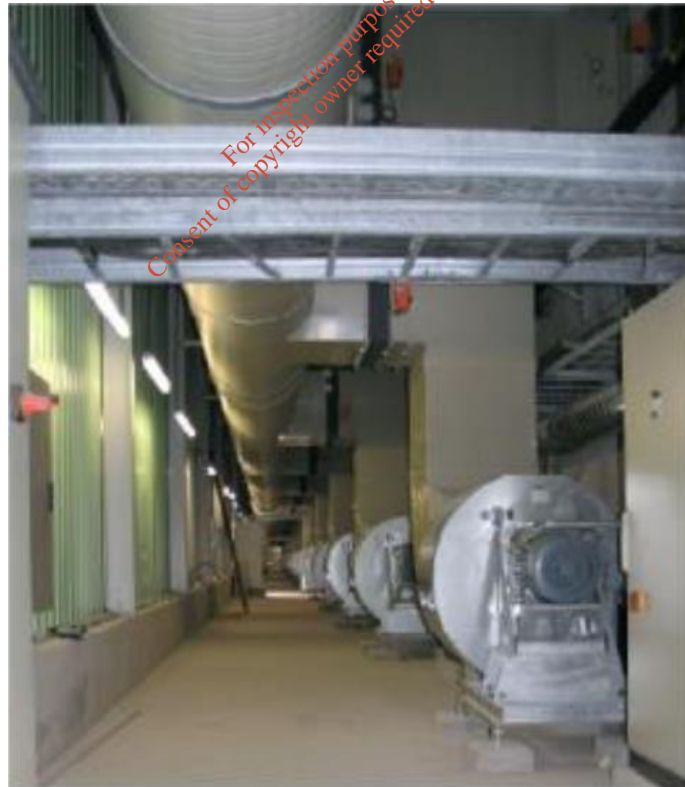
Figure 3.5: Typical Aeration Fan and Ductwork Installation
