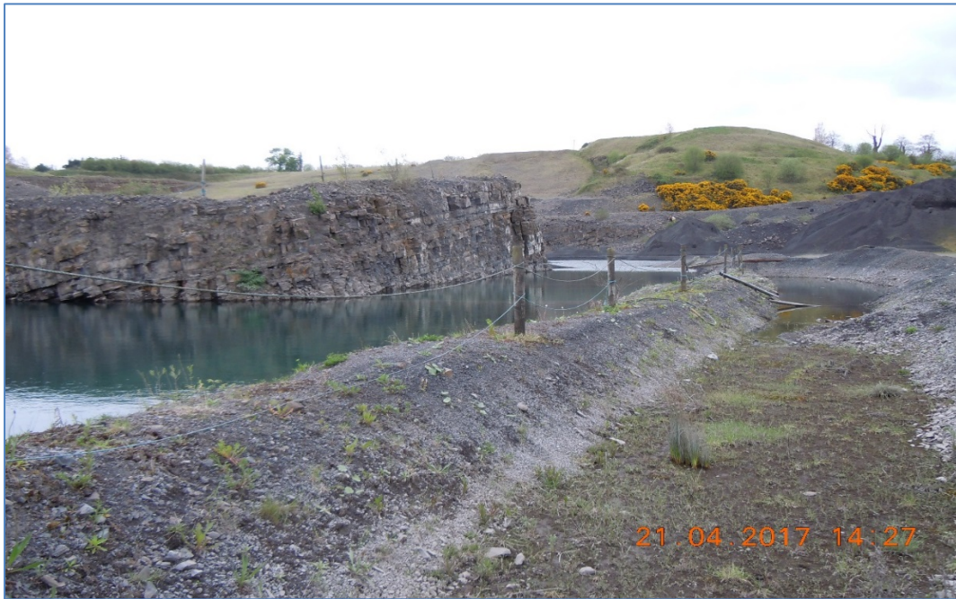
Figure 2: Groundwater on the quarry floor
