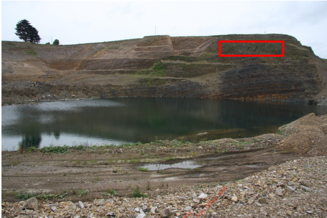
Figure 11. Proposed area for the installation of artificial or creation of natural ledges (where feasible) on the western boundary.
