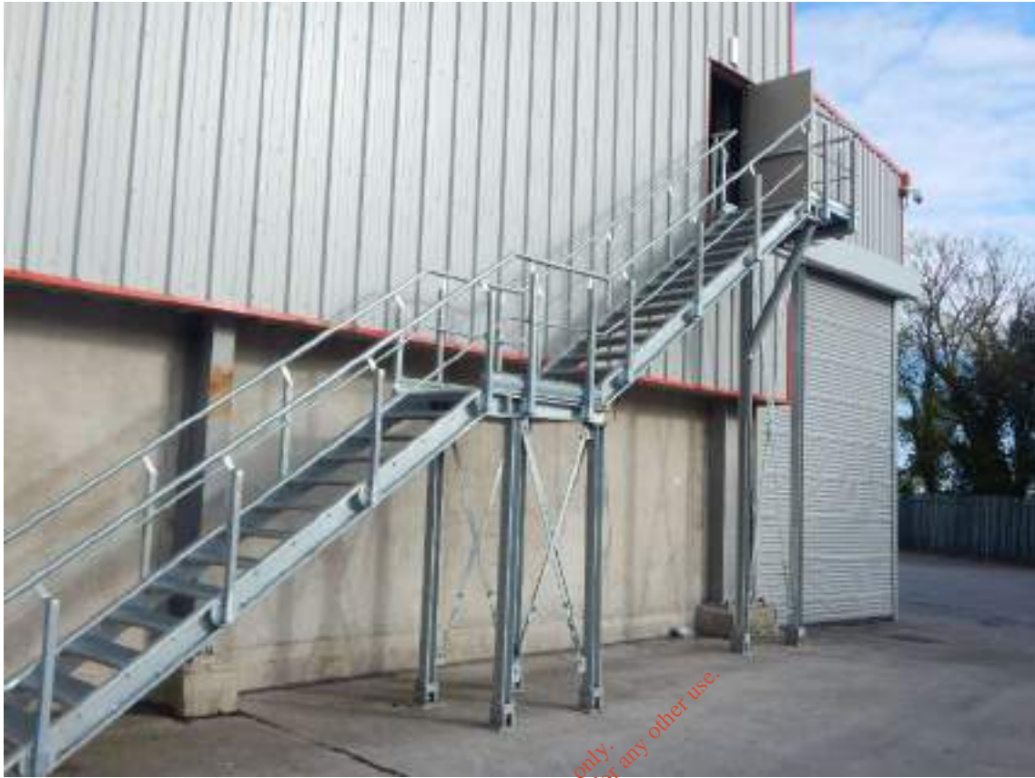
Figure 1.35: Yard Area: Emergency Exit Stairway
