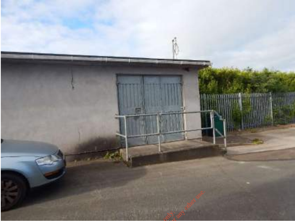
Figure 1.27: Yard Area: ESB Substation
