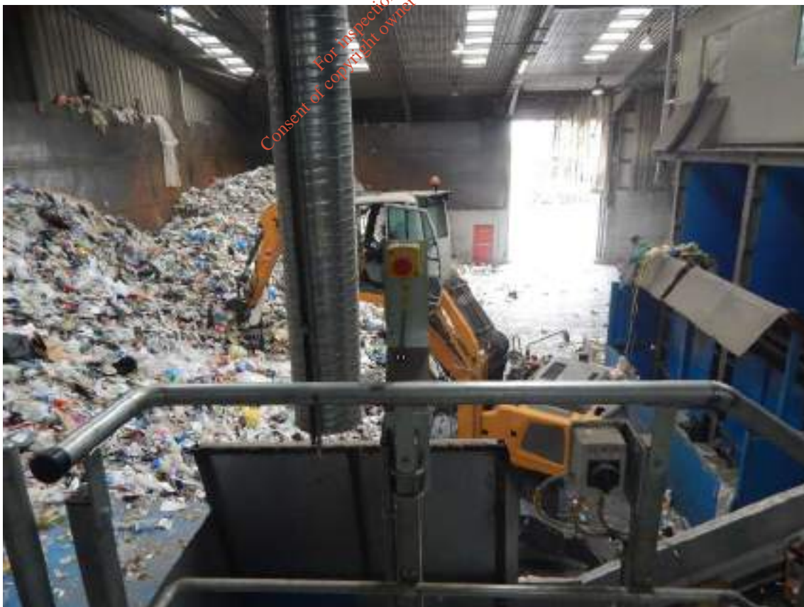
Figure 1.14: MRF Building: Emergency Stop Button
