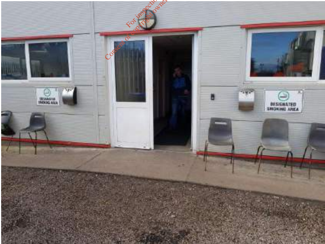
Figure 1.36: Administration Building: Designated Smoking Area outside canteen
