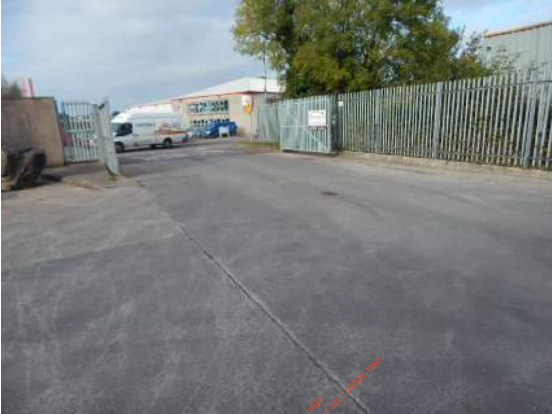
Figure 1.29: Yard Area: Exit Gate
