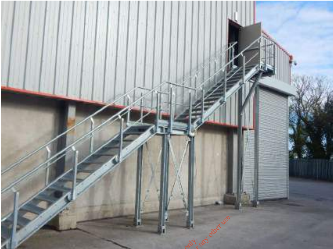
Figure 1.35: Yard Area: Emergency Exit Stairway
