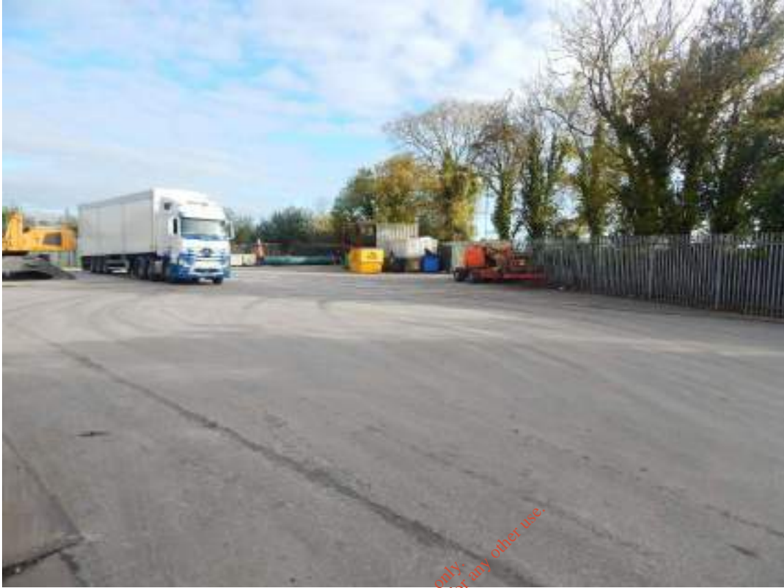
Figure 1.5: Yard Area: Rear of Site Including Workshop (Container)
