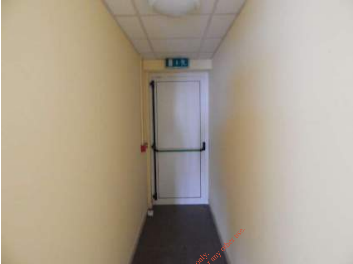
Figure 1.43: Administration Building: Push to Exit Door
