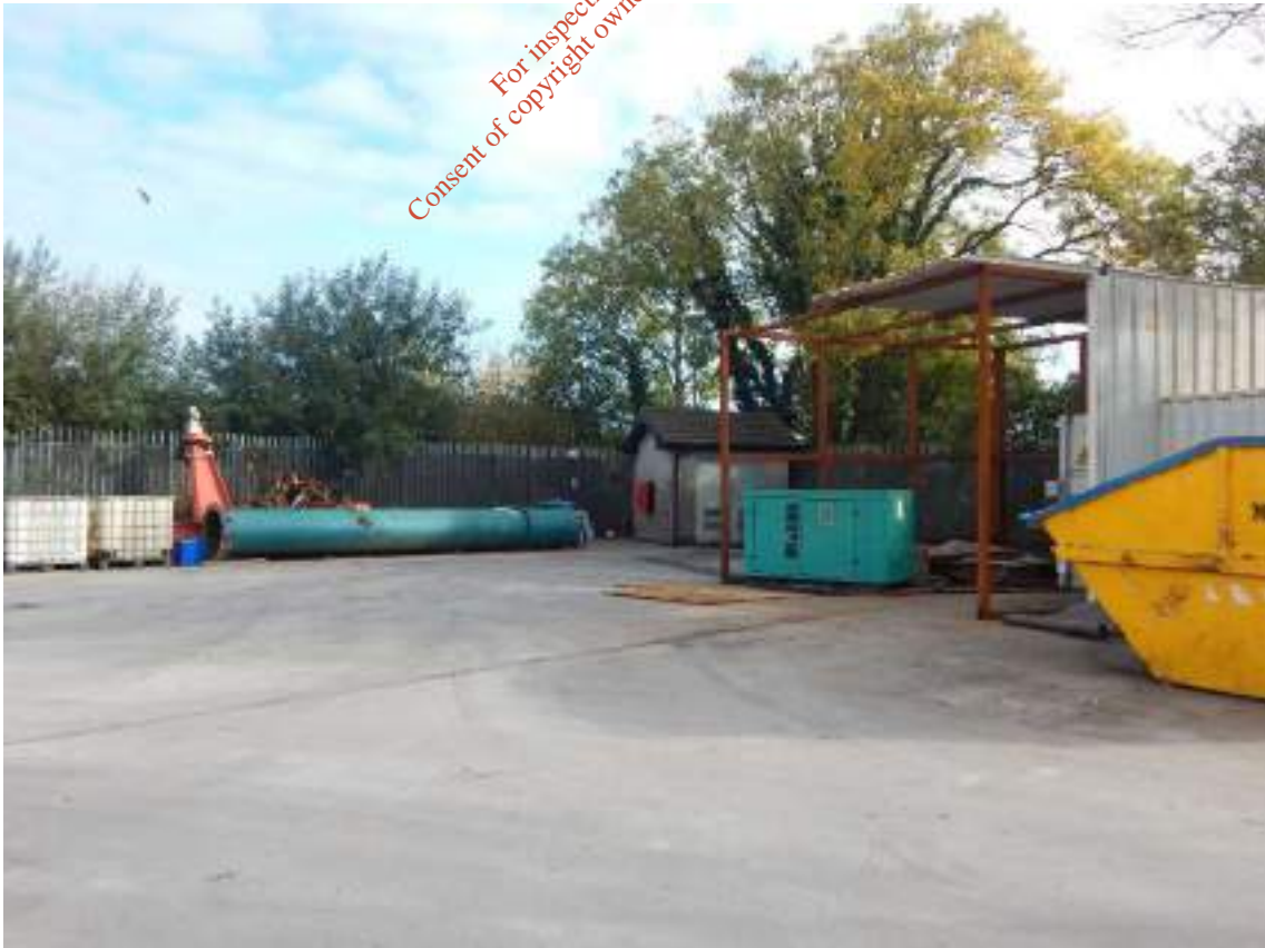
Figure 1.6: Yard Area: Oil storage Shed and Entrance to Workshop
