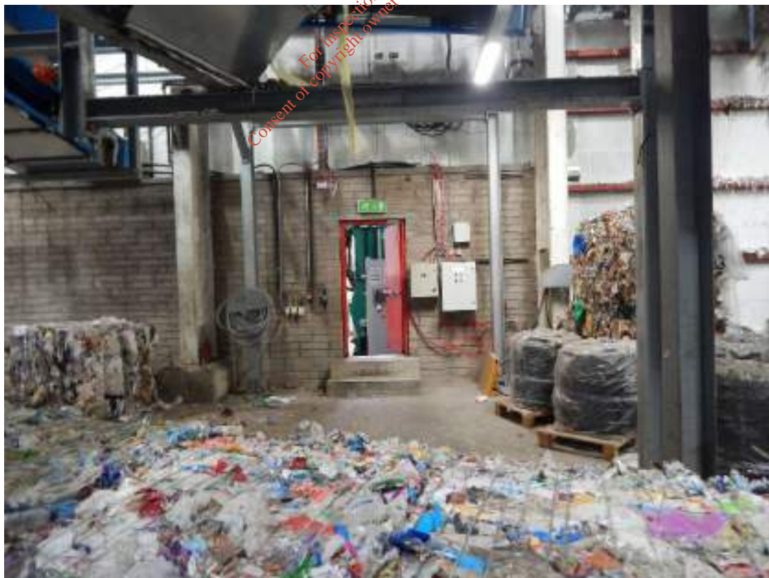
Figure 1.22: MRF Building: Emergency Exit
