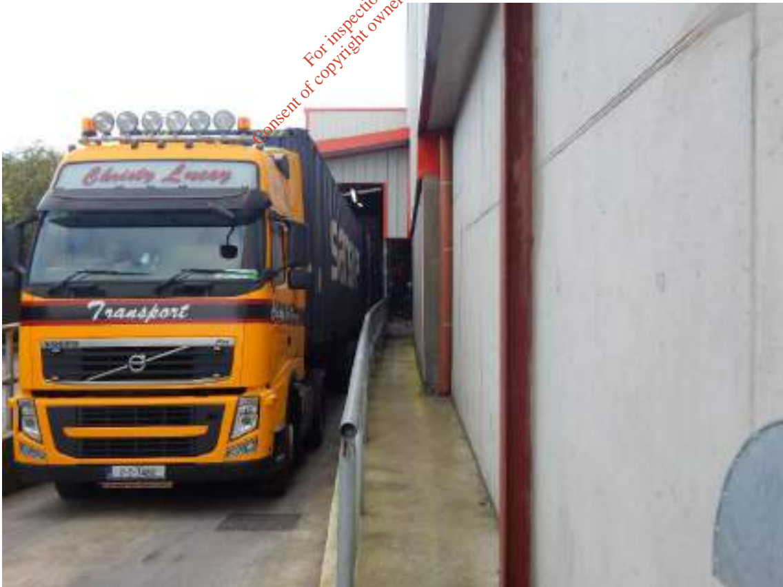
Figure 1.28: Yard Area: Docking Bay Ramp
