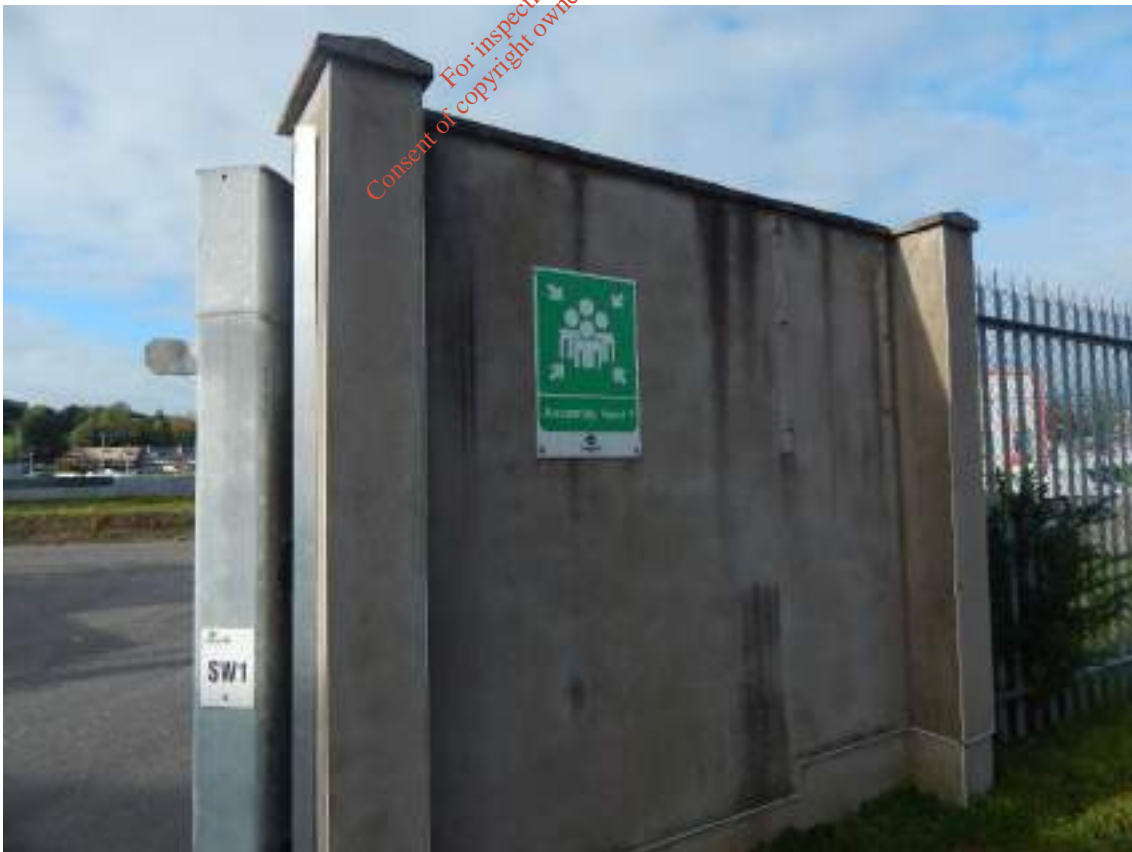
Figure 1.4: Yard Area: Fire Assembly Point by Entrance
