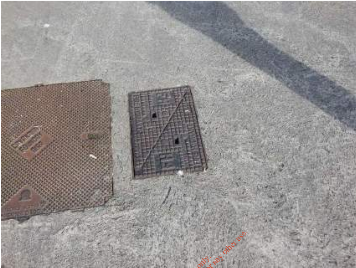
Figure 1.31: Yard Area: Hydrant 1 by Exit
