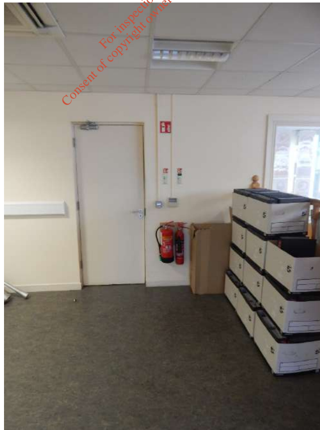
Figure 1.40: Administration Building: Fire Extinguishers
