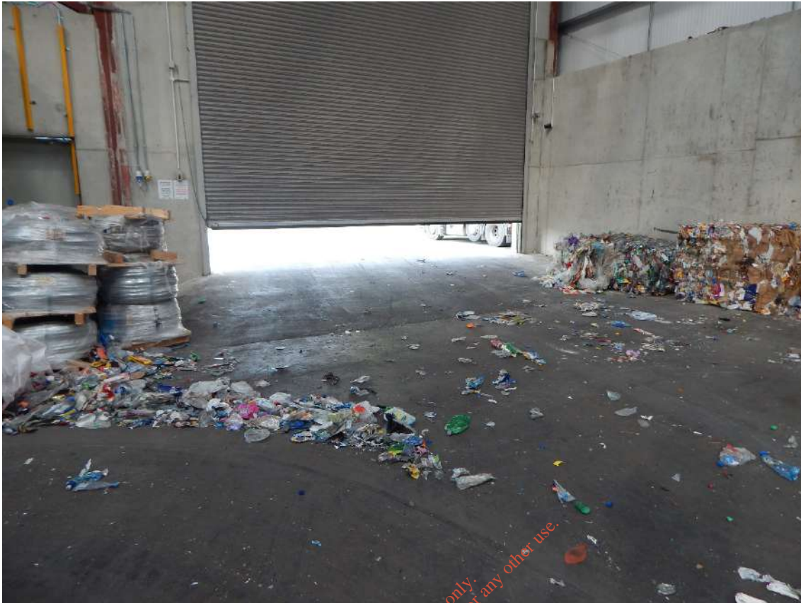
Figure 1.25: MRF Building: Fire Water Retention Ramp into and Out of MRF Building
