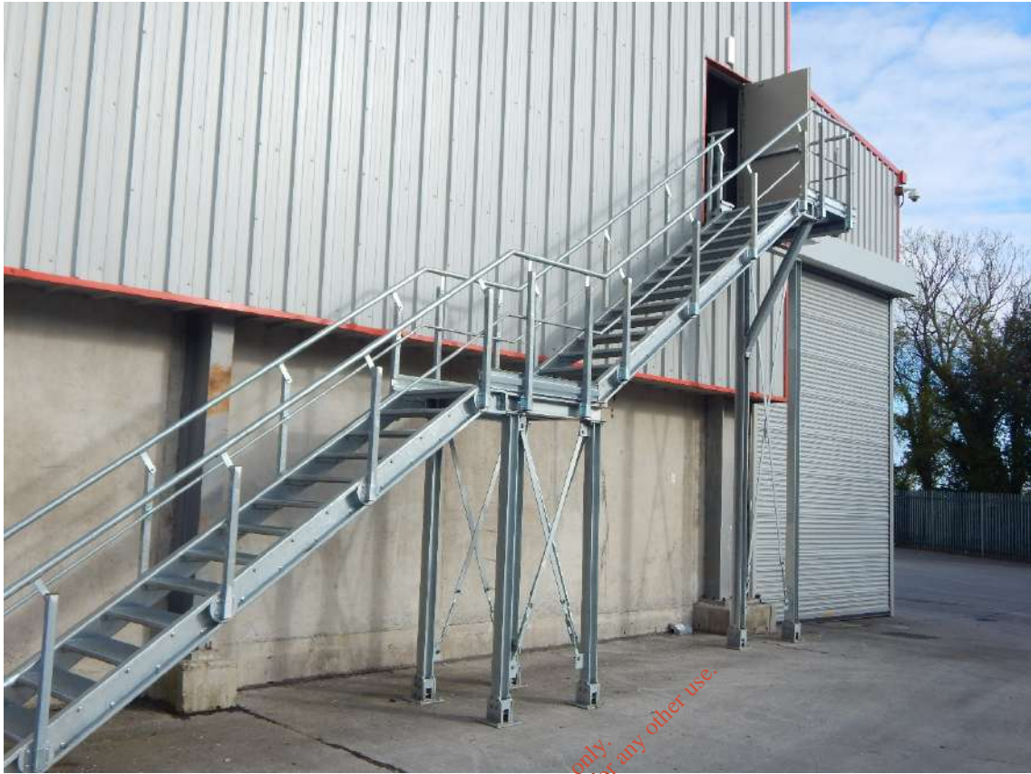
Figure 1.35: Yard Area: Emergency Exit Stairway
