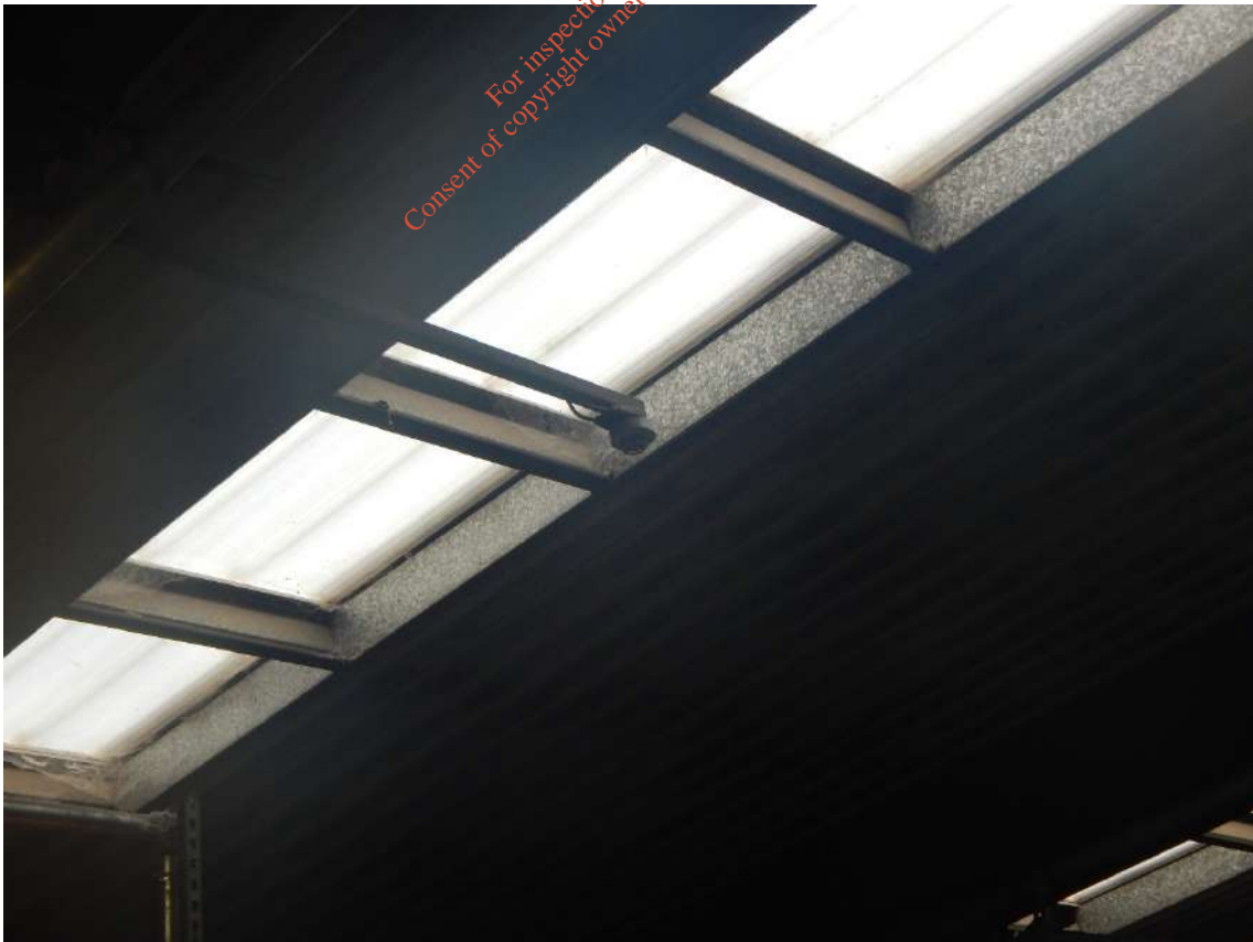
Figure 1.16: MRF Building: Smoke Detector
