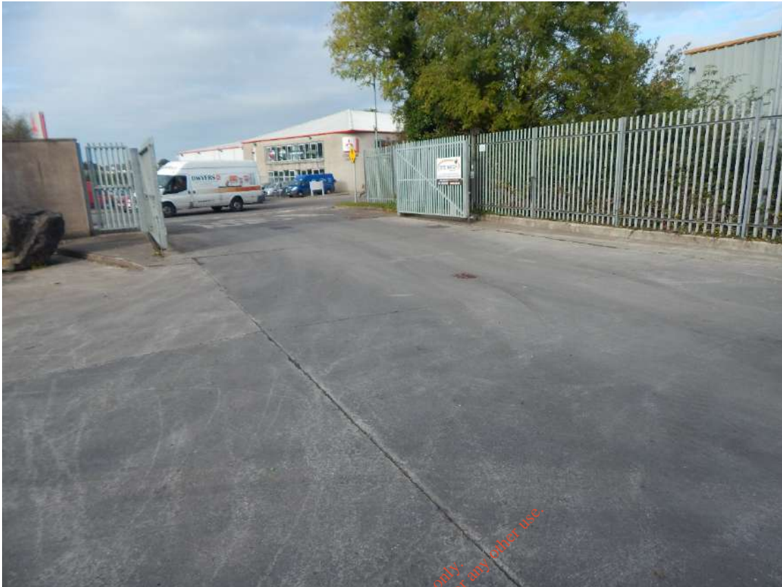
Figure 1.29: Yard Area: Exit Gate
