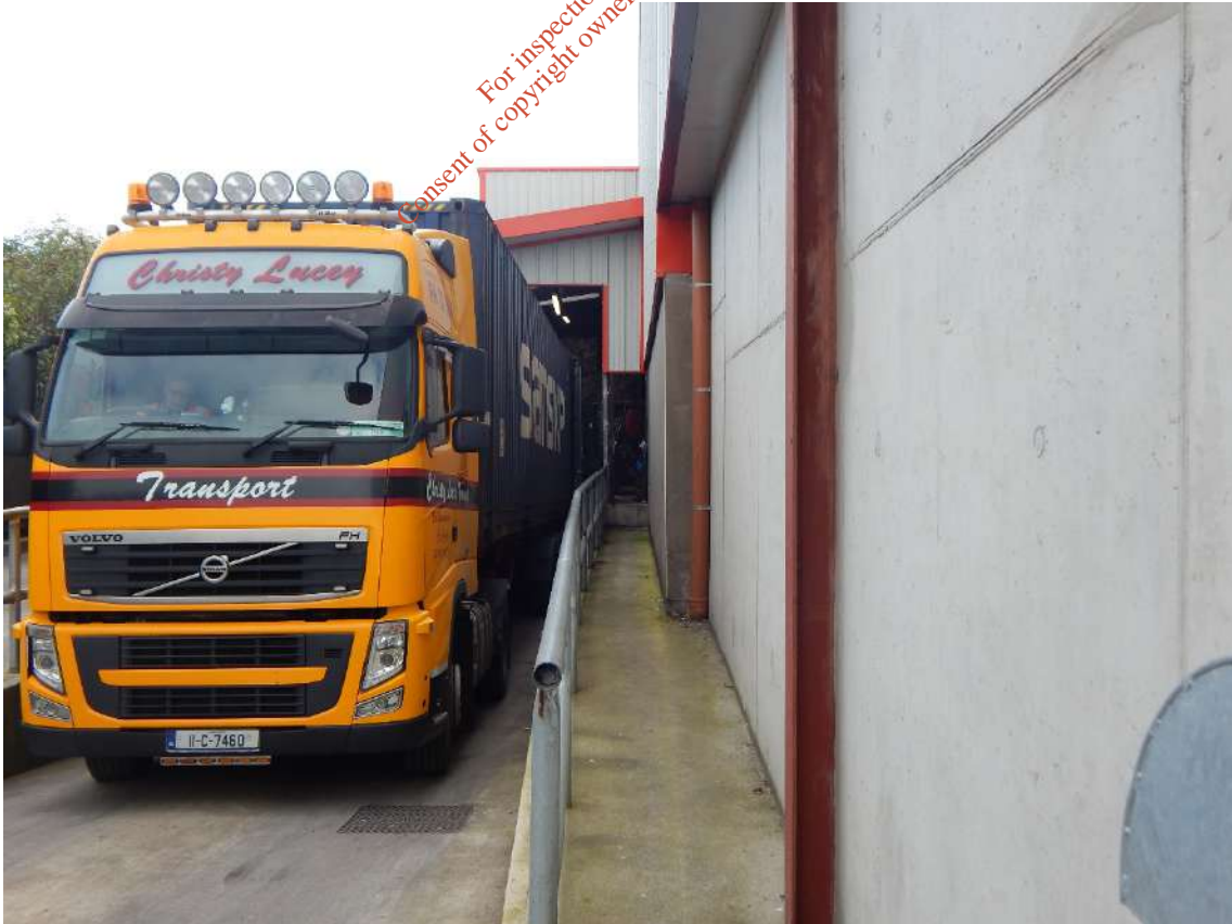
Figure 1.28: Yard Area: Docking Bay Ramp
