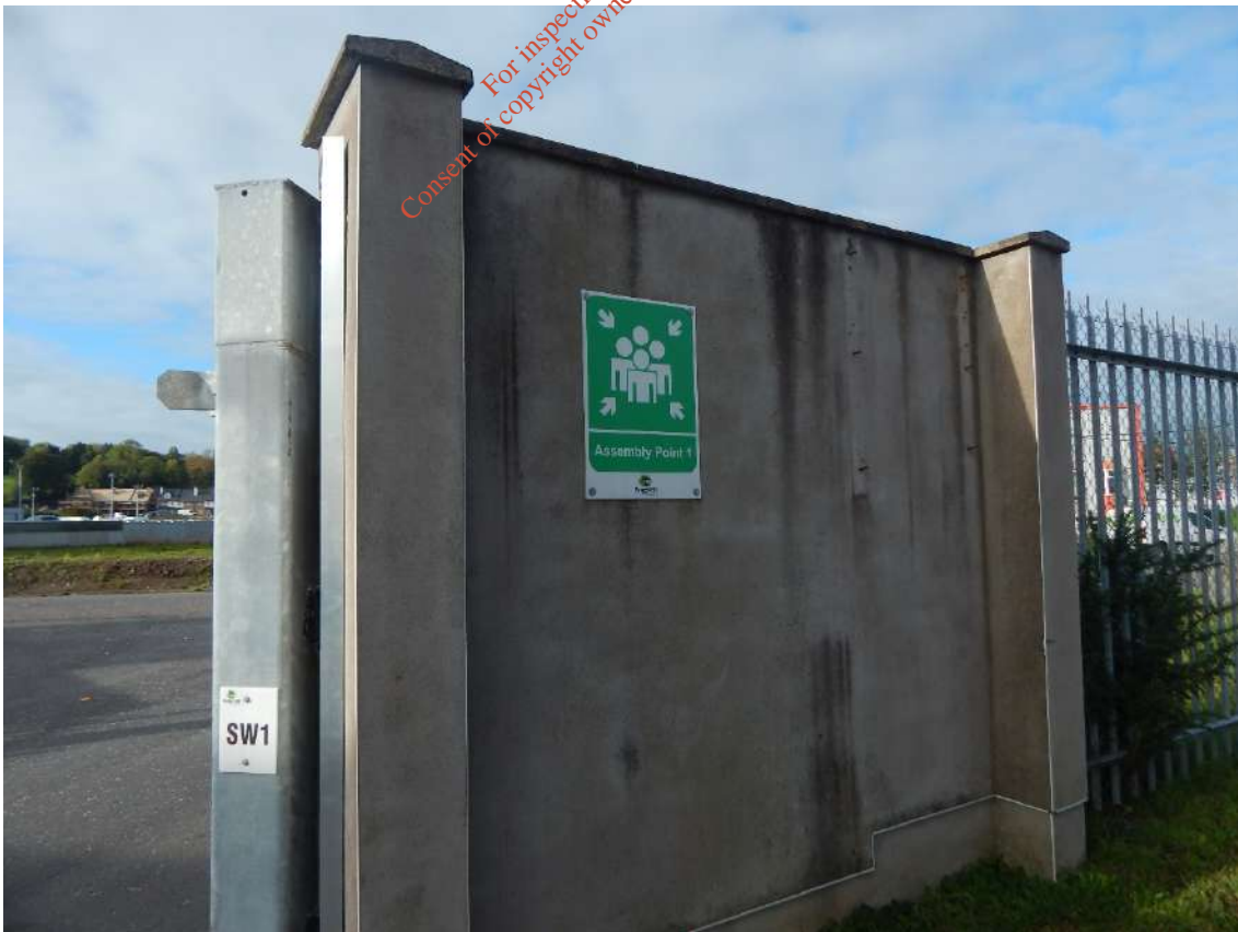
Figure 1.4: Yard Area: Fire Assembly Point by Entrance
