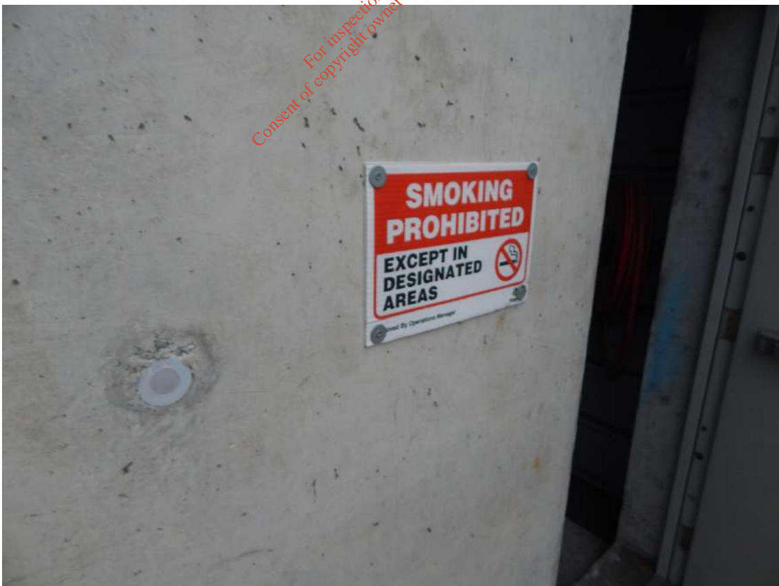
Figure 1.26: Yard Area: No Smoking Sign
