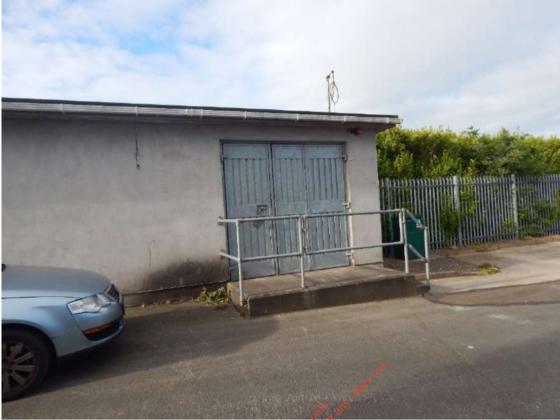
Figure 1.27: Yard Area: ESB Substation
