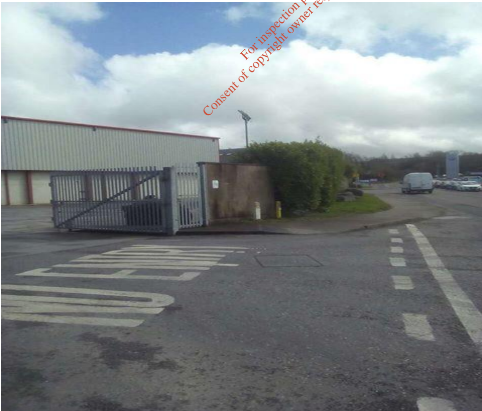
Photograph 4 Screening at Road Frontage
