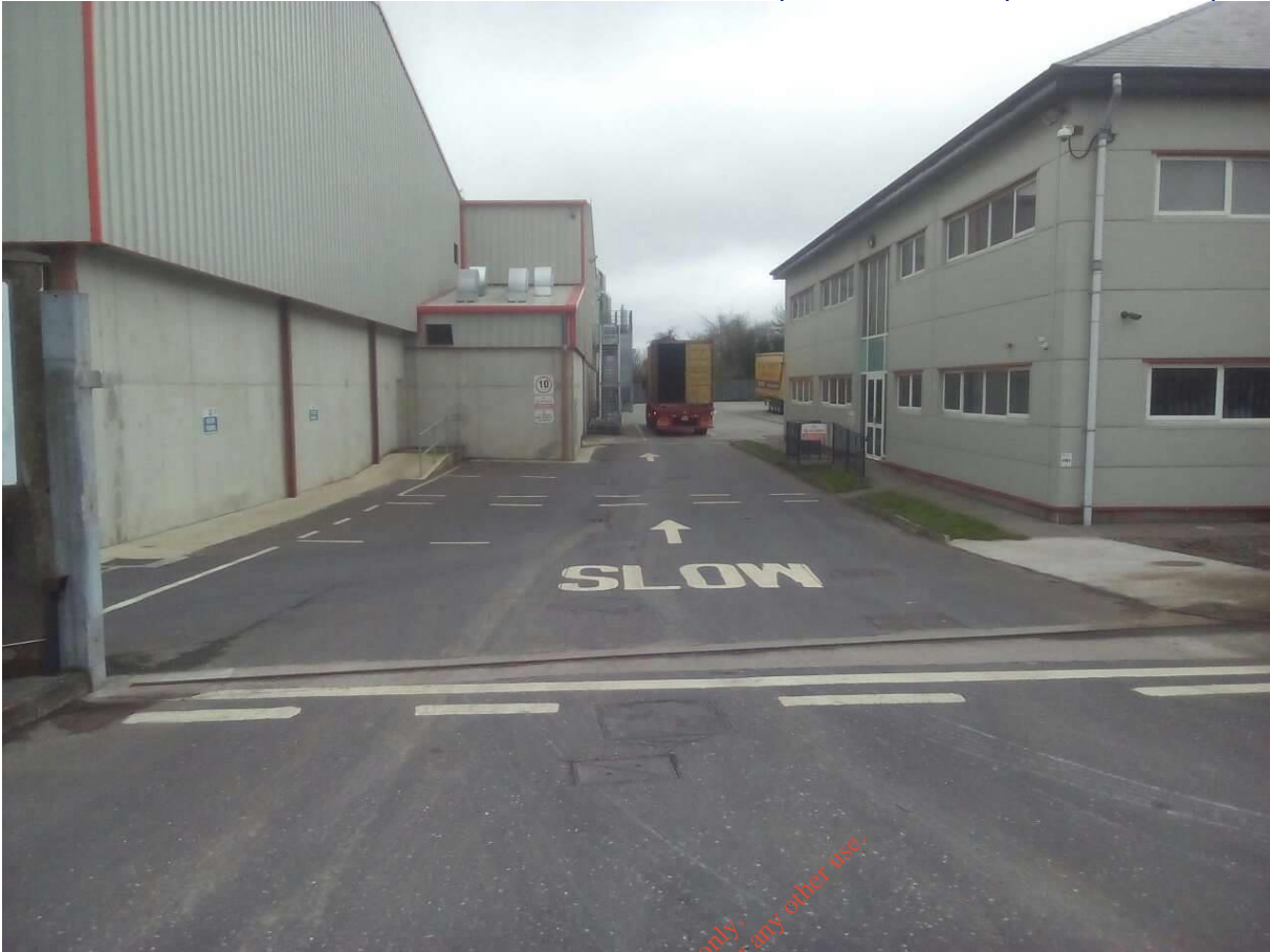
Photograph 3 Southern Entrance, Offices to the Right and Processing Building to the Left
