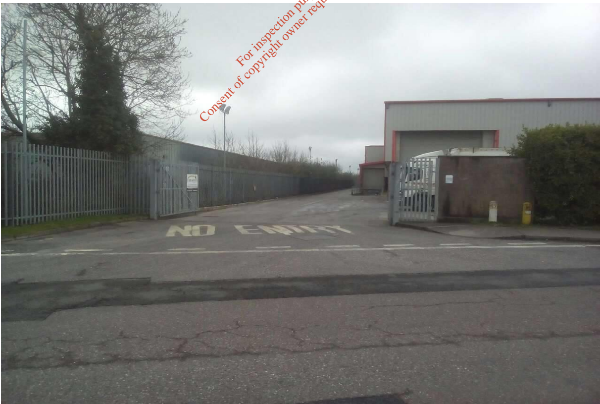
Photograph 2 Northern Entrance and North Western Elevation of Process Building
