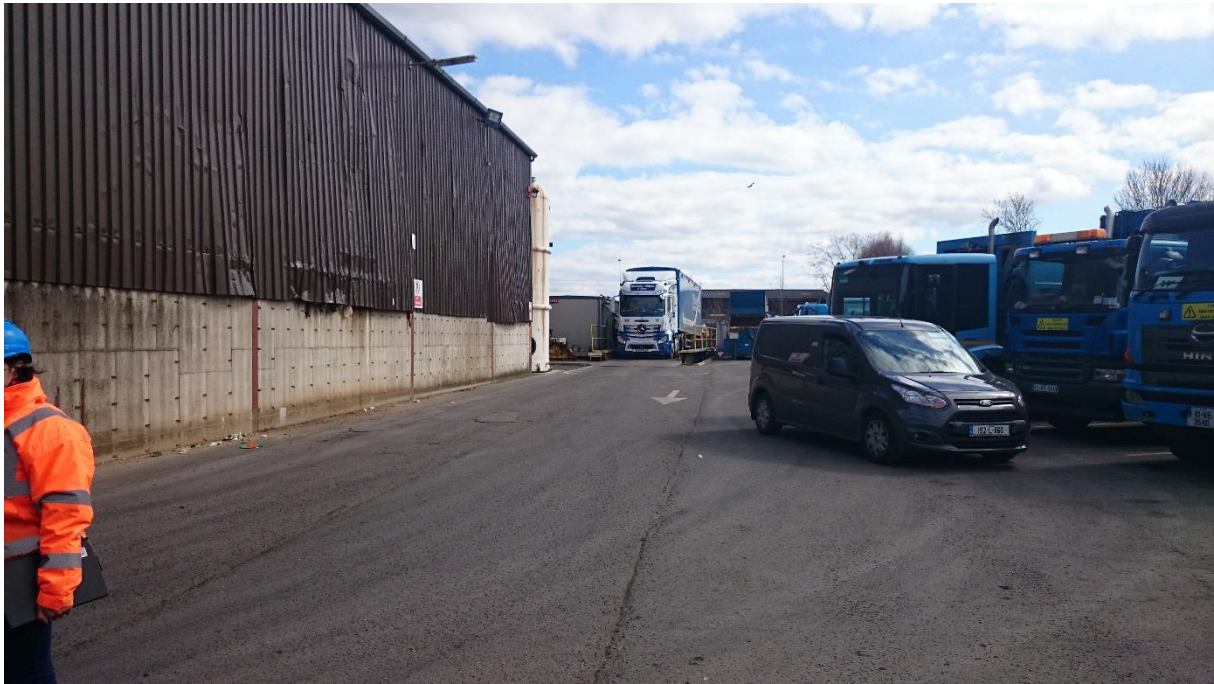
Photograph 5 Internal Access Road and Western Elevation of Main Processing Building
