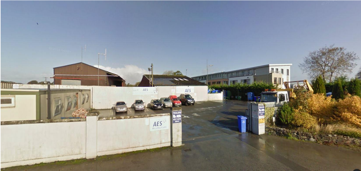
Photograph 1 Southern Boundary: Entrance to Civic Amenity Area
