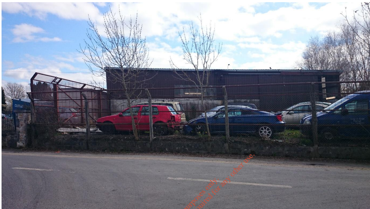
Photograph 7 Commercial Unit to the South of the Facility
