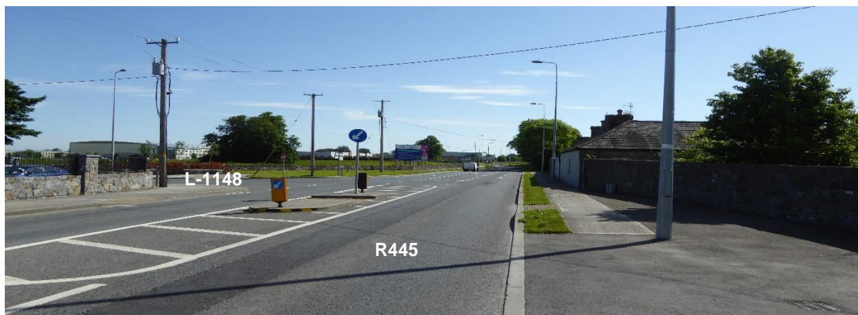
Image 4 – Eastbound on the R445 towards the priority junction with the L-1148, Junction 3
