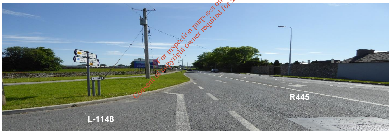
Image 5 – Junction 3 visibility to the east from the L-1148
