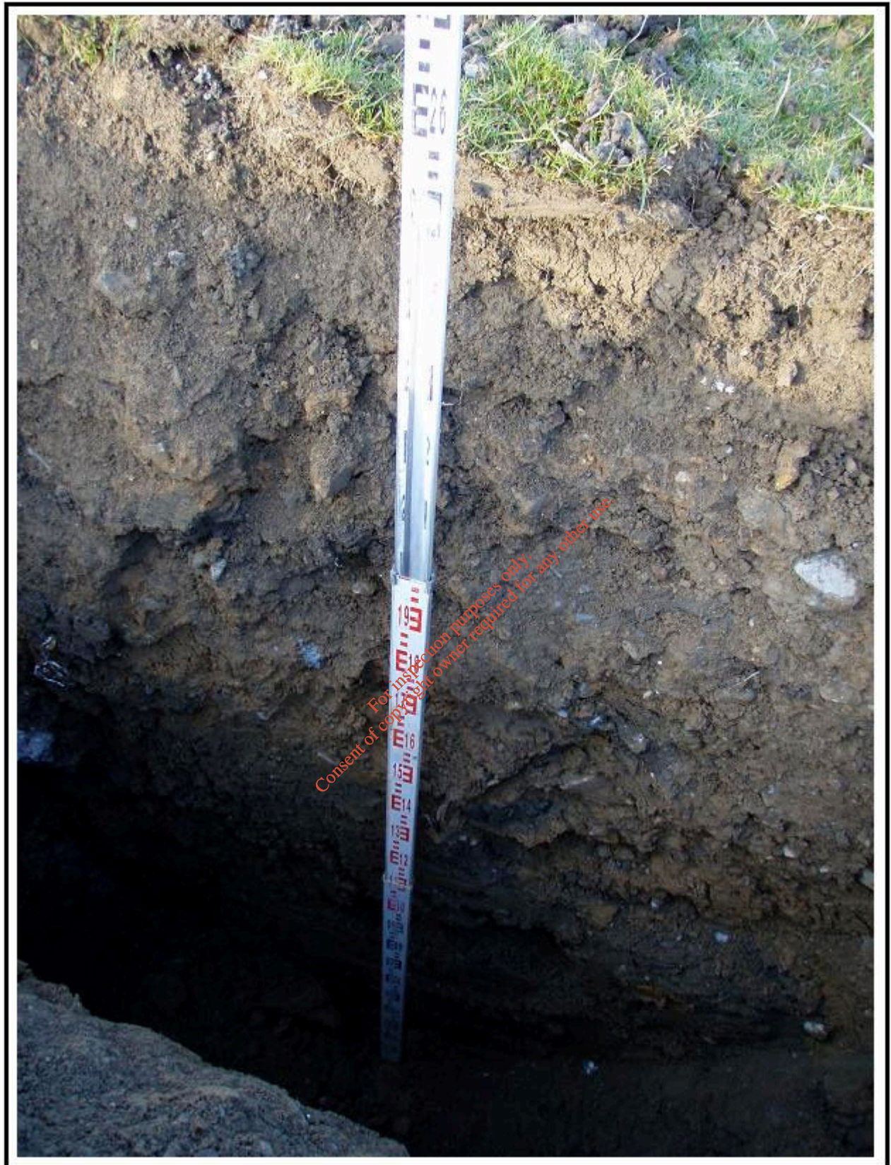
Plate A5: Profile of shallow topsoil overlying subsoil in trial hole no. 5. See the occasional concrete pieces and fragments of steel within the profile and the well aerated nature of the material, with no groundwater seepages recorded to 2.47m depth.
