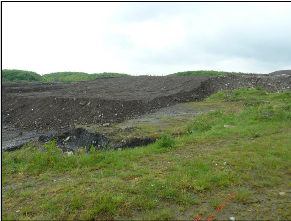
Plate 4.9-2 Area P2, looking south, prior to backfilling
