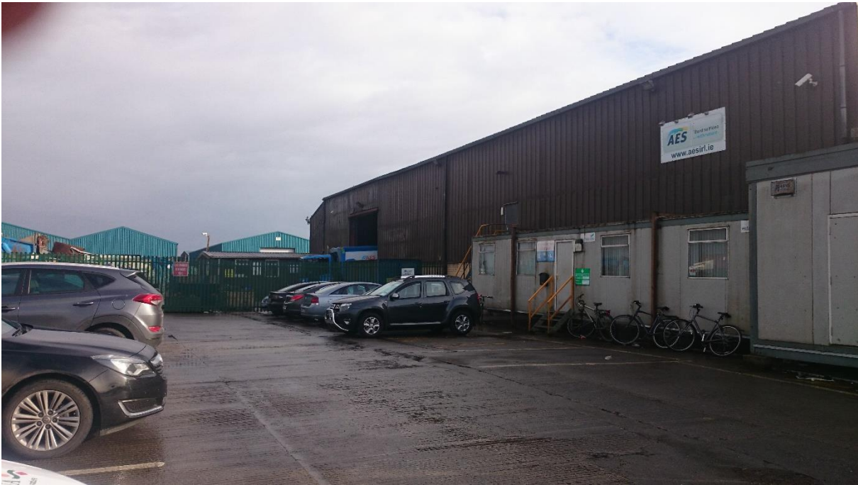
Photograph 1 Northern Elevation of Process Building and Offices
