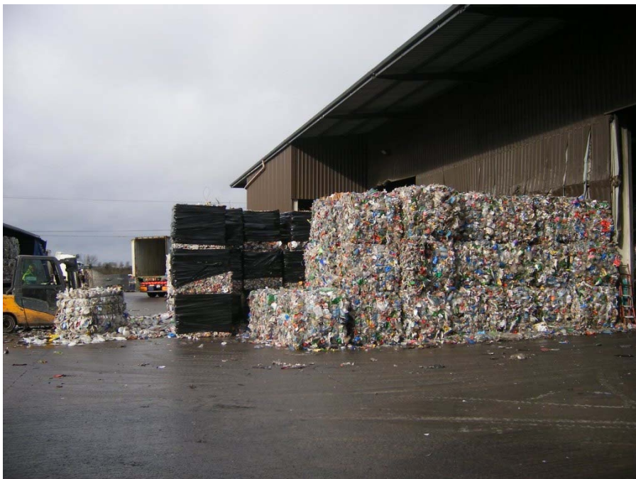
Figure 2.8: Canopy area over bale storage
