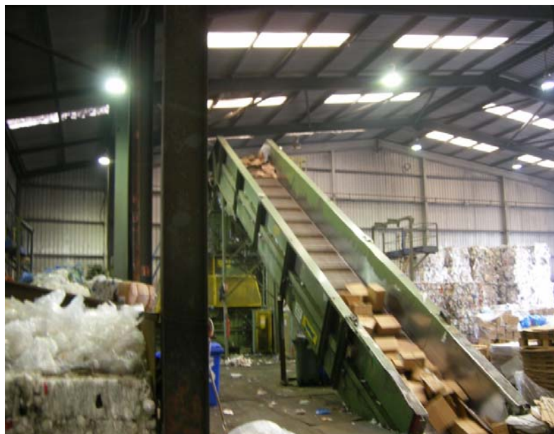
Figure 2.4: Baling Plant area
