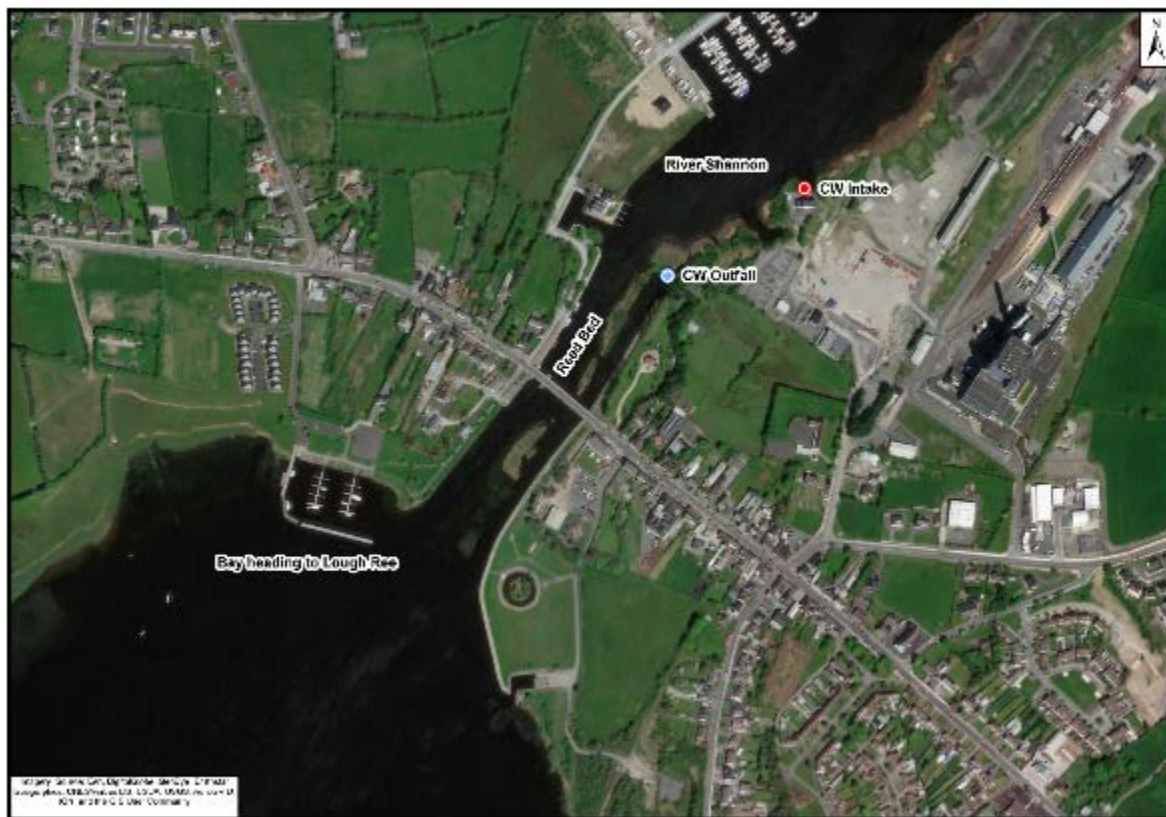
Figure 3-1. River Shannon at Lanesborough
