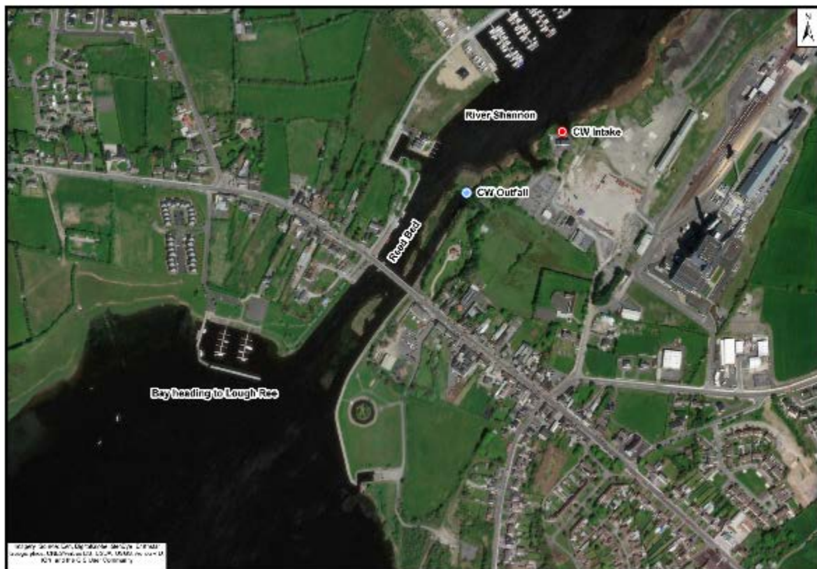
Figure 2-1 River Shannon at Lanesborough
