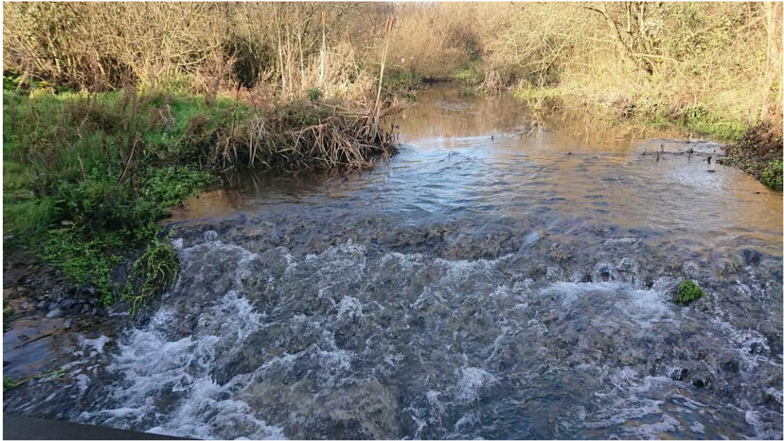
Plate 3 Tramore River: Site C – view upstream from crump weir (15-12-2017).
