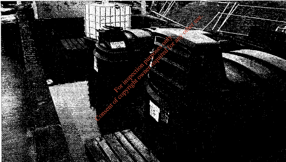
Photo 2 – Green Diesel and Waste Oil Tanks
