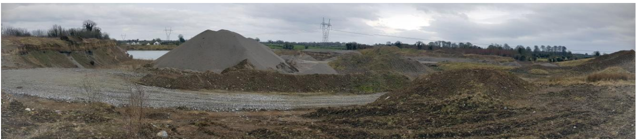
Plate11-4: Panoramic view of the application area looking east.
