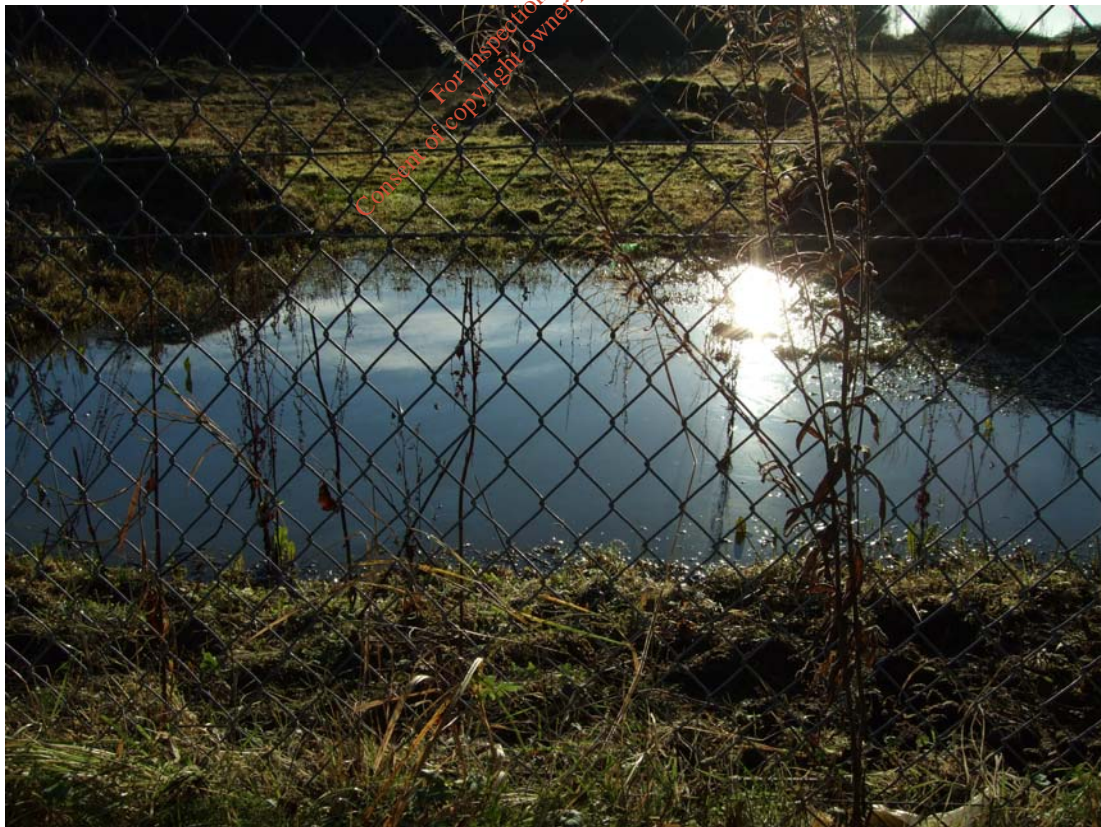
Photo 8: Area of ponding inside northern boundary fence.
