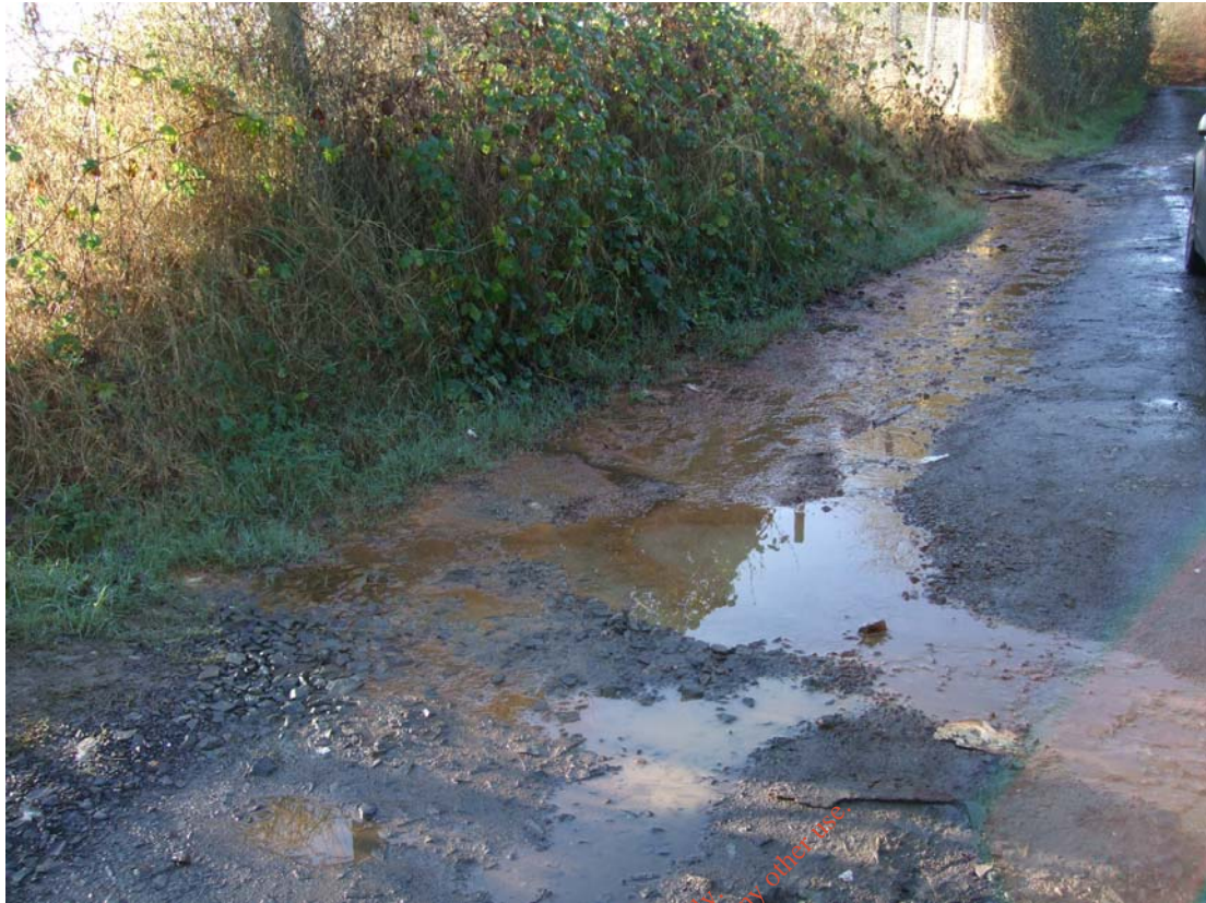
Photo 9: Leachate runoff onto road from inside northern boundary.
