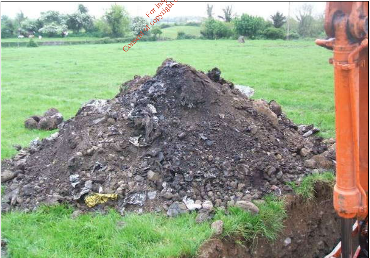
Photograph No 2 Waste material encountered in TP-6
