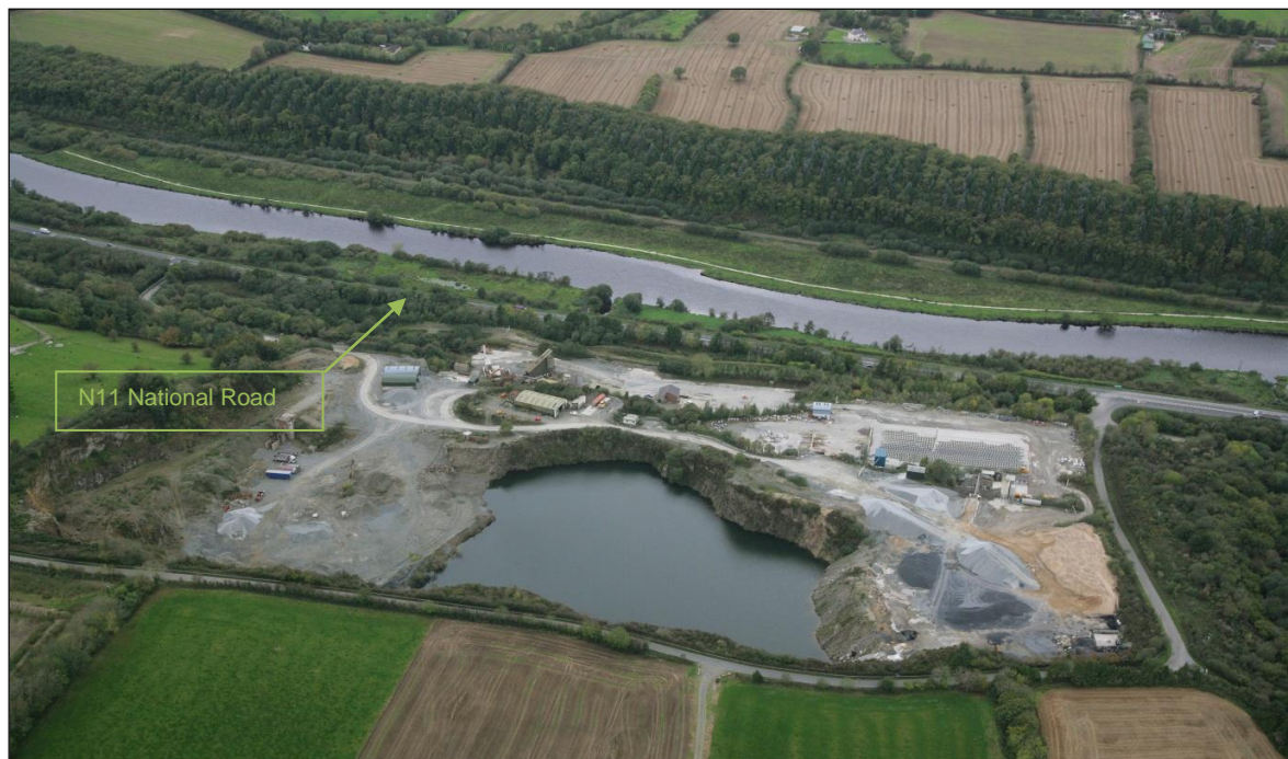
Figure 3 Oblique Aerial View of Existing Quarry
