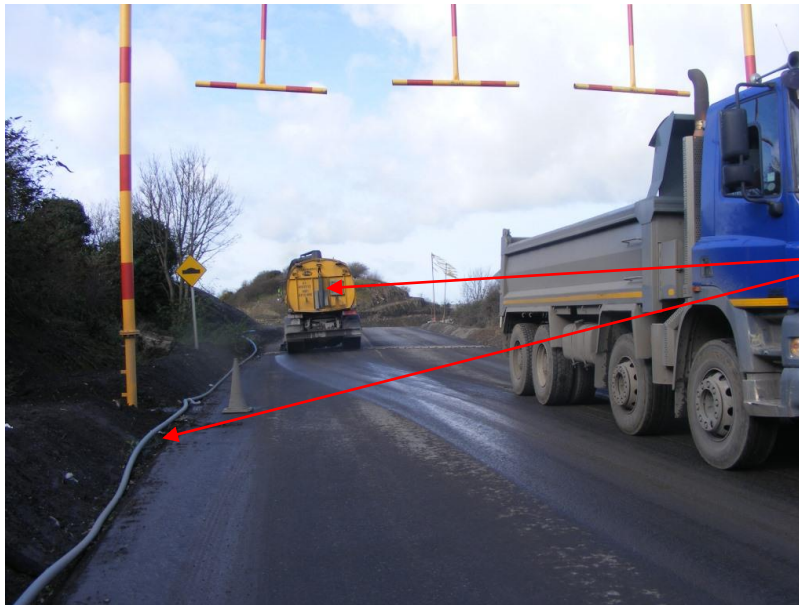
Plate 2 – Road Sweeper and Sprinklers under Construction
