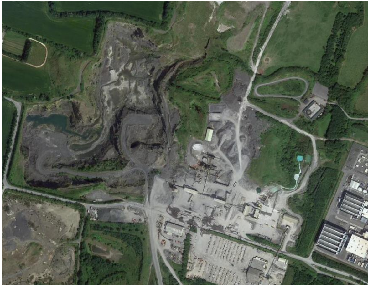
Plate 1 Aerial View of Site from Google Earth (July 2013)
