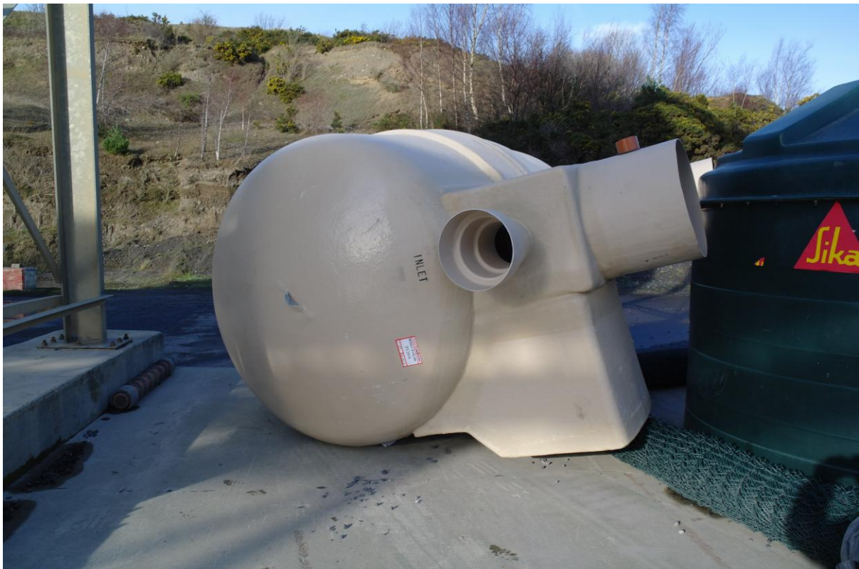
Photo 6 – Hydrocarbon Interceptor Awaiting Installation
