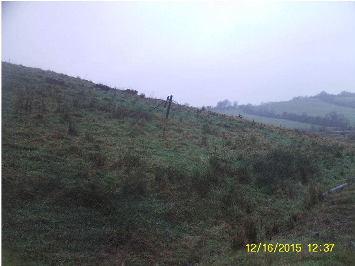
Figure 13 – Northeast Slope of Cell 3 (facing northwest)
