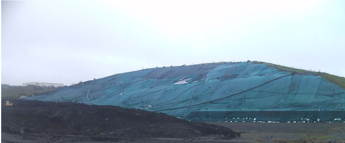
Figure 16 – North Slope of Cell 4 (facing southeast)
