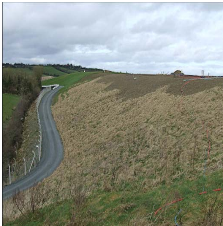
Figure 8 – Northwest Slope of Cell 1 in 2008 (facing northwest)
