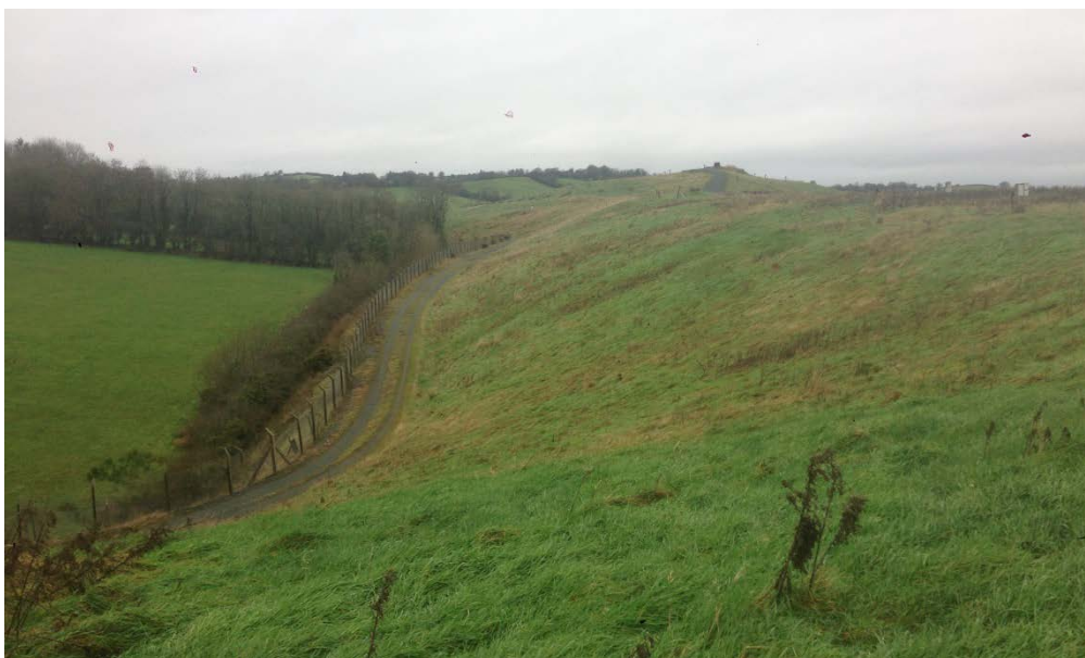
Figure 10 – Northwest Slope of Cell 1 in 2015 (facing northwest)
