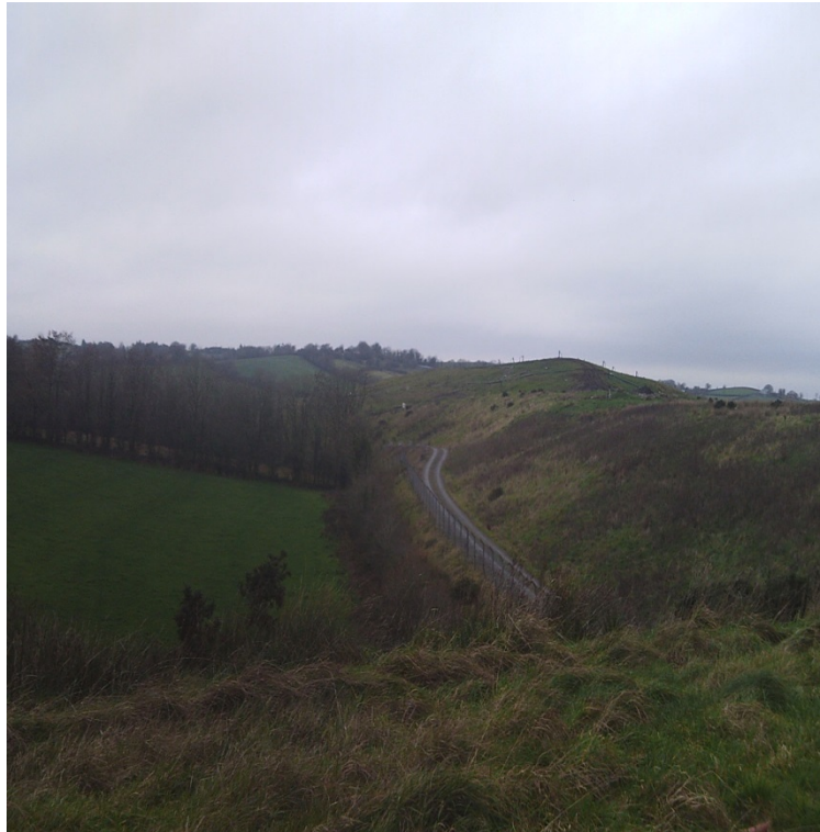
Figure 9 – Northwest Slope of Cell 1 in 2013 (facing northwest)
