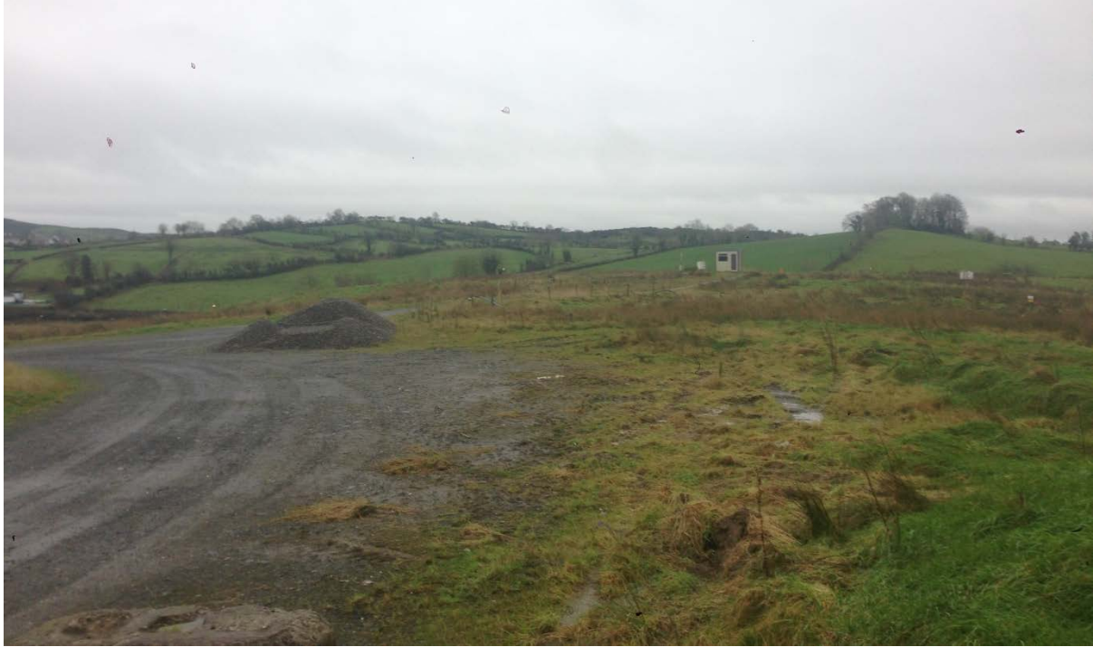
Figure 18 – Crest of Landfill (facing southeast)
