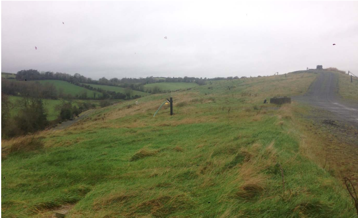
Figure 19 – Crest of Landfill (facing northwest)
