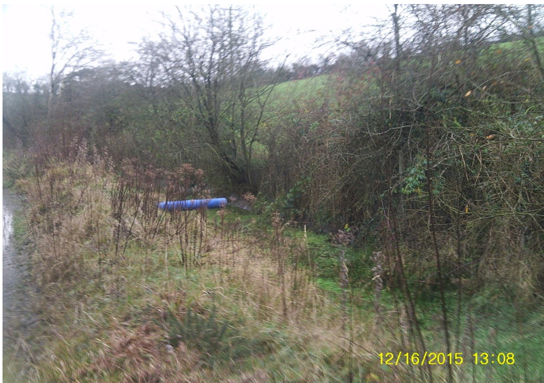
Figure 4 – Ponding in channel at the toe of the Southwest Slope of Cell 0 (facing southwest)
