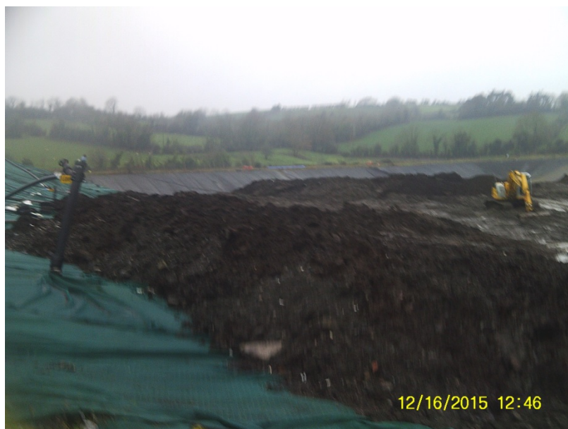
Figure 17 – Topsoil in Cell 4 (facing west)
