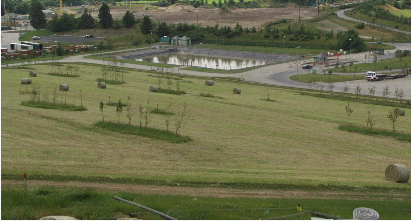
Figure 2-1: Completed Landfill Cap at Arthurstown
