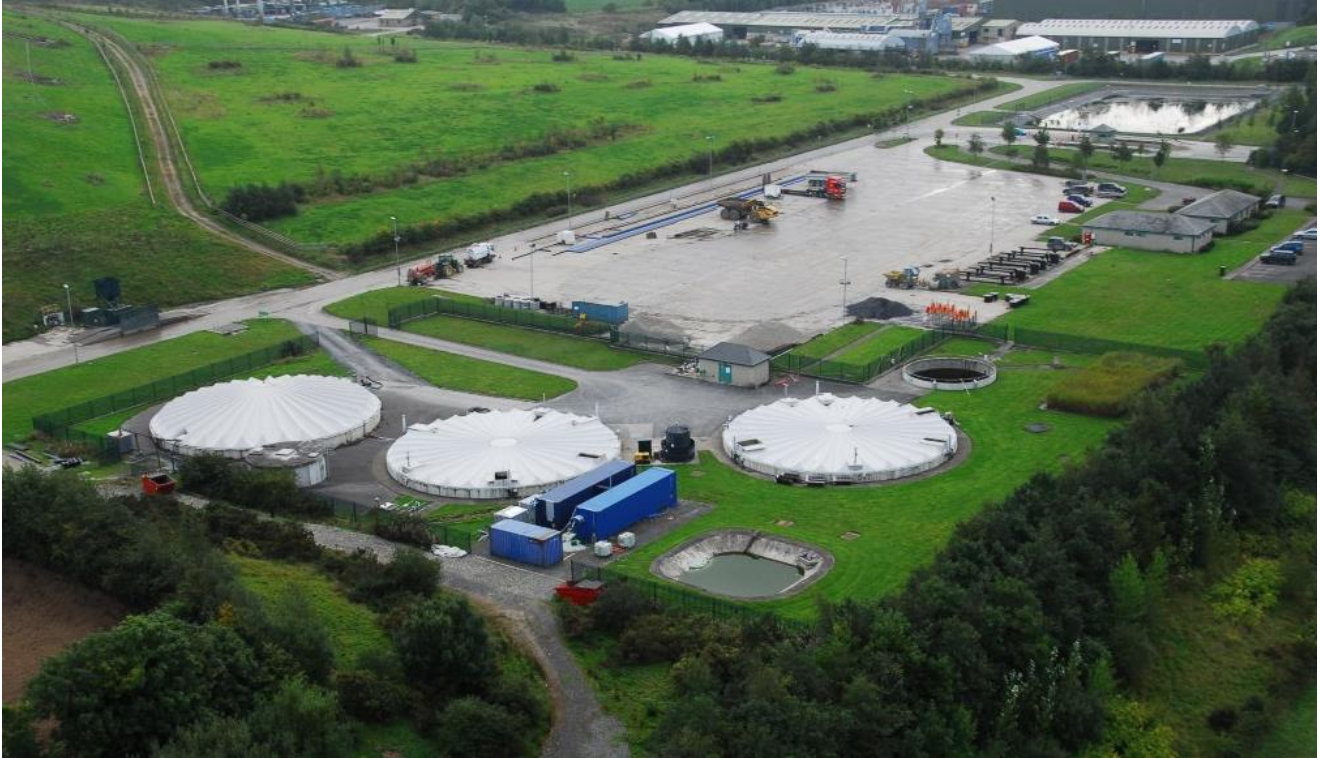
Figure 4-1: Leachate Treatment Plant
