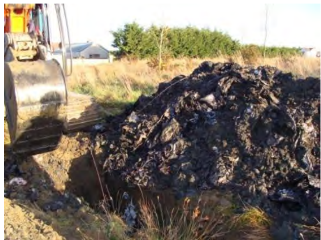
Figure 1.19: Waste removed Trial Pit 10
