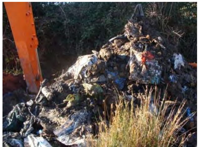
Figure 1.12: Waste removed Trial Pit 6
