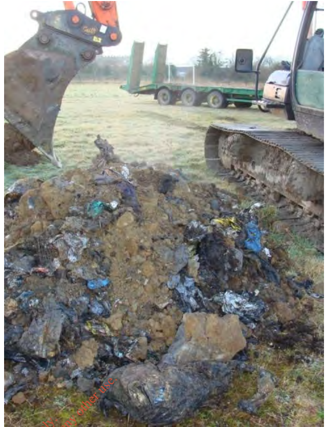
Figure 1.5: Waste removed Trial Pit 1
