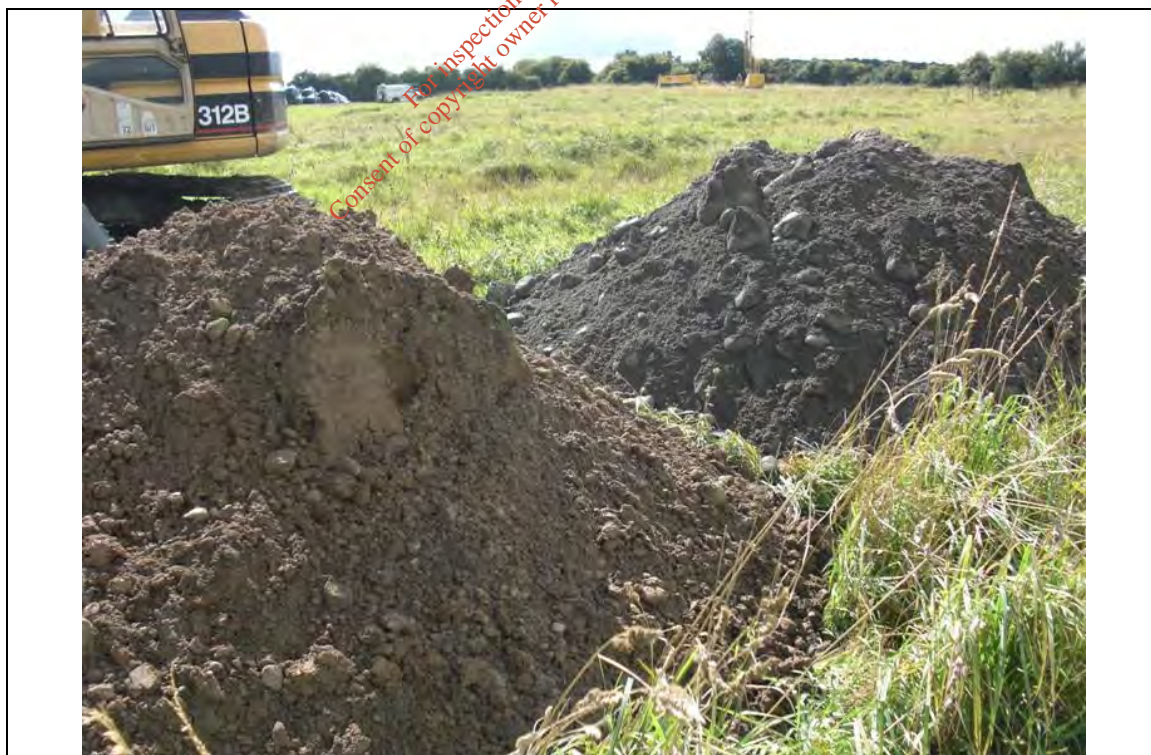
Photograph No: 4 Natural clays and gravels at location TP01.
