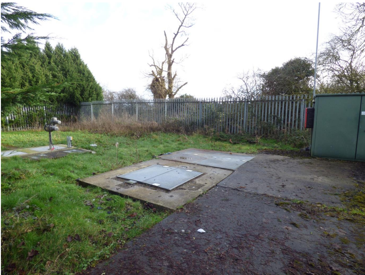
Figure 2: Moulden Bridge Pumping Station Rathoath
