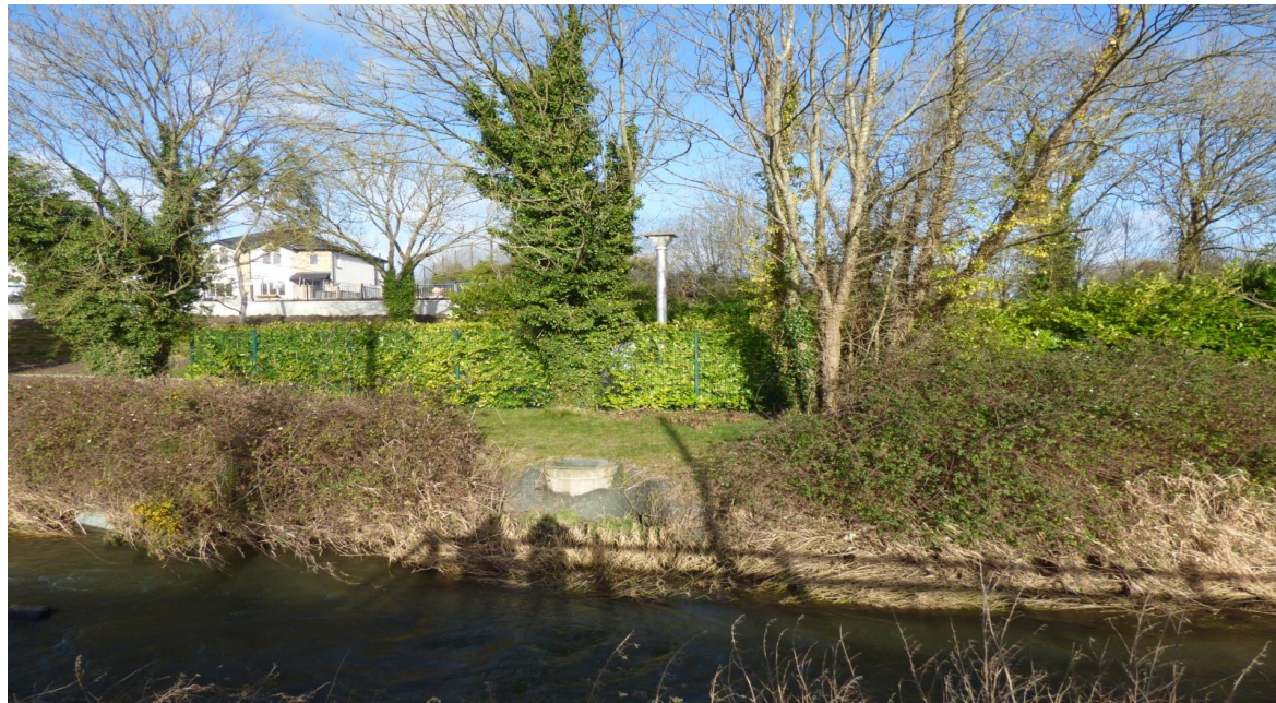
Figure 1: Picture of Milltown Pumping Station and the River Broadmeadow
