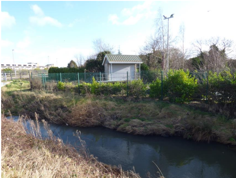
Figure 1 Castle Street Pumping Station
