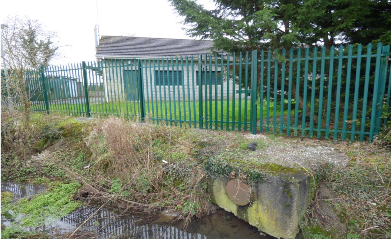
Figure 1: Emergency Overflow Point from Kilbride Pumping Station
