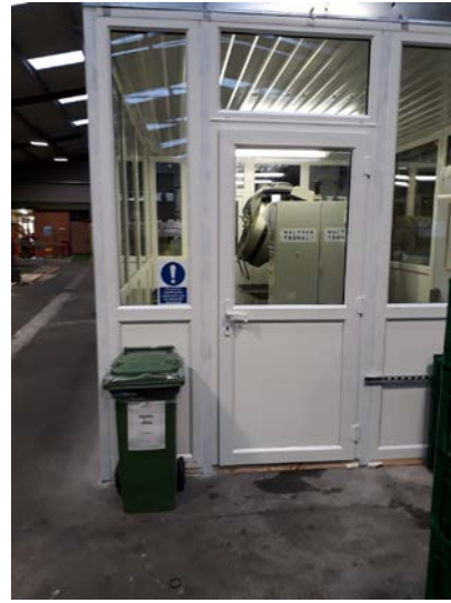
Fig.2 Small extension containing new enclosed rotary drum unit for Gleitmo coating process.
