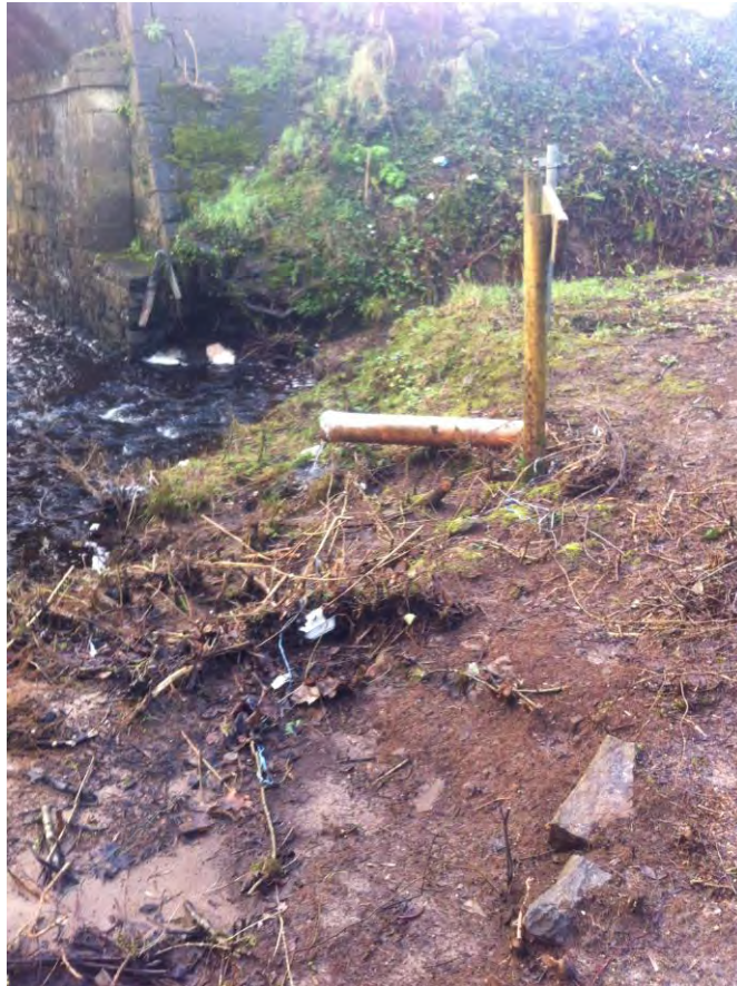
Photograph 8: Surface Water Discharge at SW1
