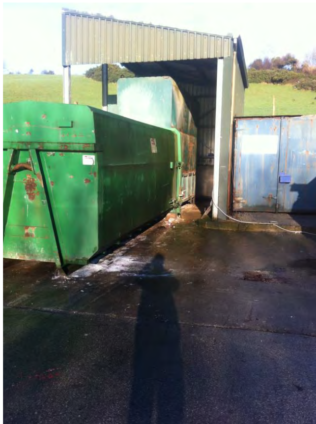
Photograph 4: Compactor Unit with associated Road Gully.
