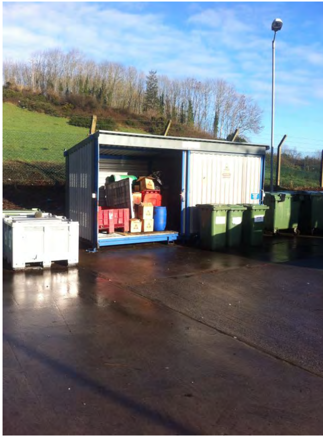
Photograph 3: Bunded and Covered ChemStore for Haz Waste Storage.
